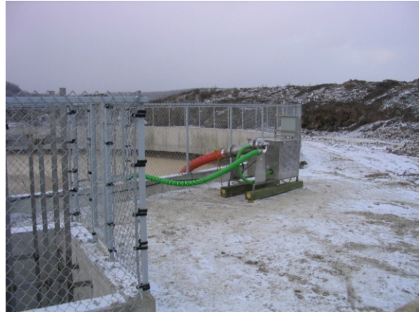
Showing Shore-mounted SAR™ Aerator
