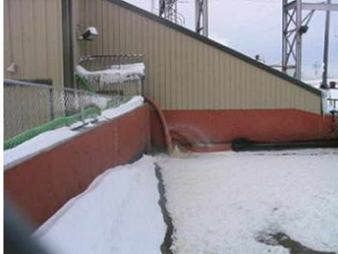
Holding Lagoon – green & brown hoses are input & output of the 250gpm Aerator
