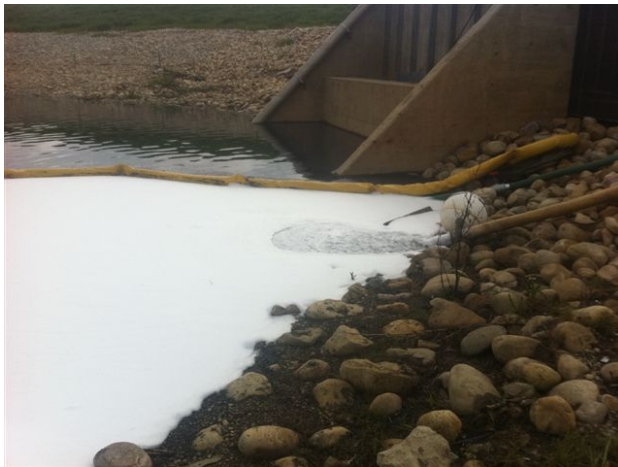
The Froth Cap pushing out the boom and covering the area inside the boom
