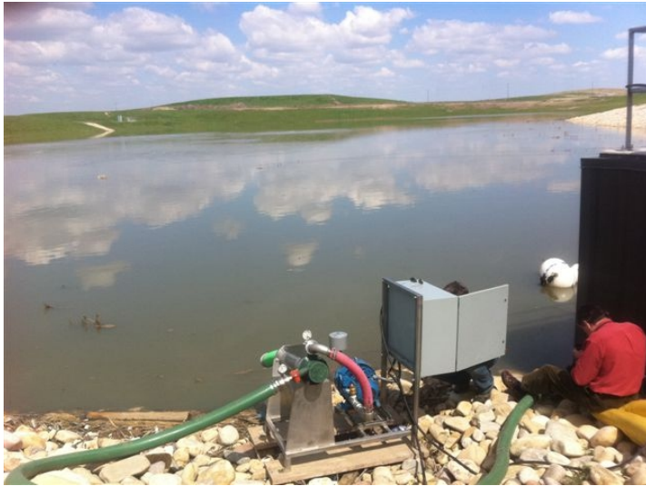
Hydro Processing's Aerator being installed at Calgary Airport pond
