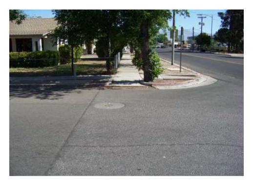
Photo #5: At Main Street looking north with US Highway 70 in the background; existing sidewalk and Sidewalk Ramps to be removed and replaced.
