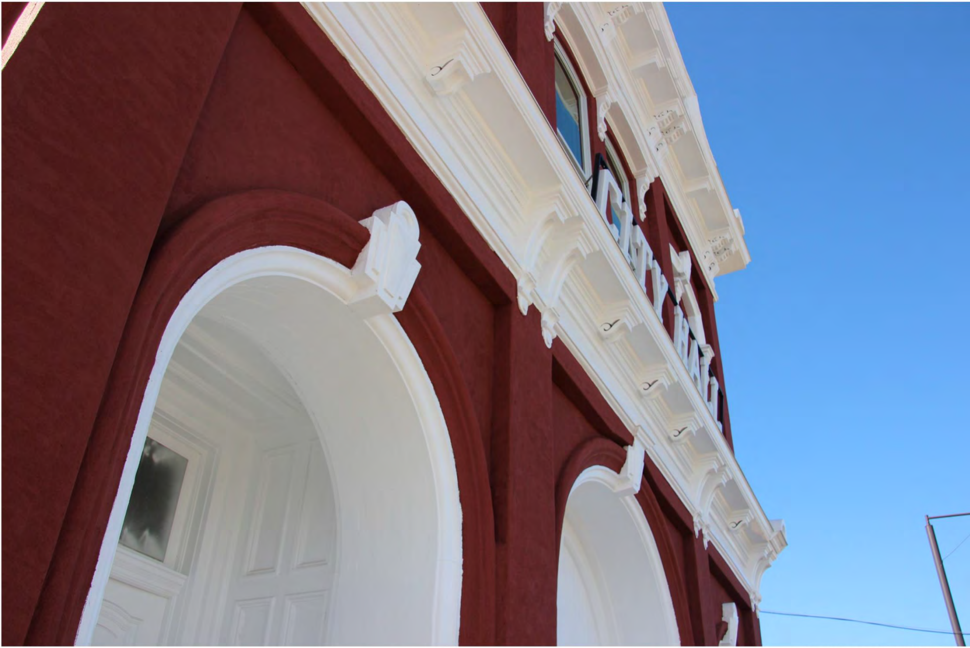
Portal Detail | After
