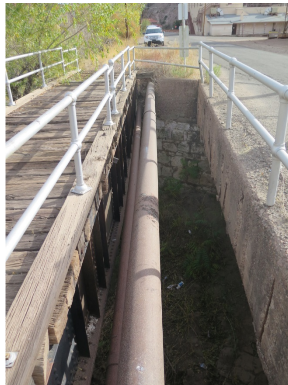
Top view of the two pipes between bridges.
