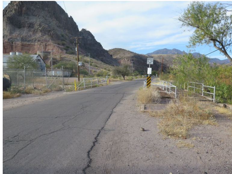
Approach Roadway – Looking North.
