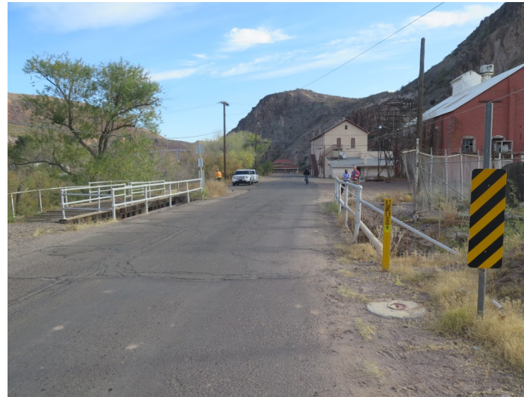
Approach Roadway – Looking South.
