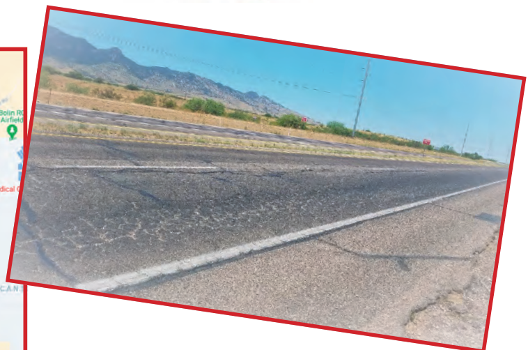
Buffalo Solider Trail disintegrating roadway surface
