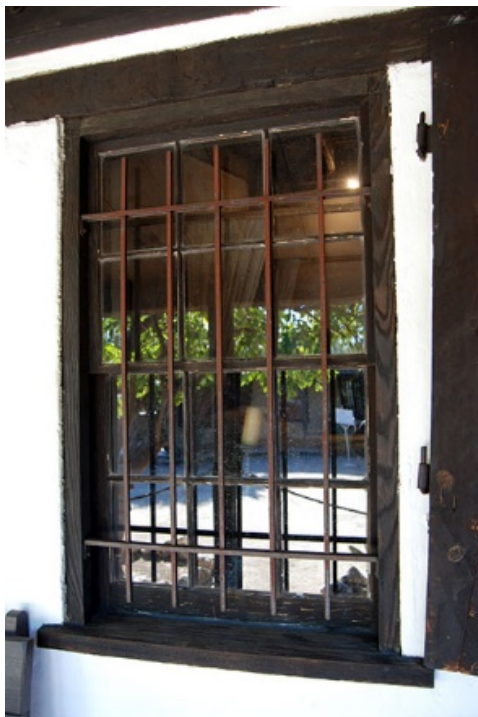
Figure 5: Typical wood window frame, sash, and trim.
