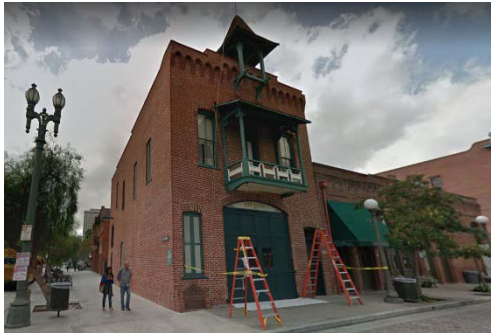
North and east façades of the Plaza Firehouse; view to the southwest.
