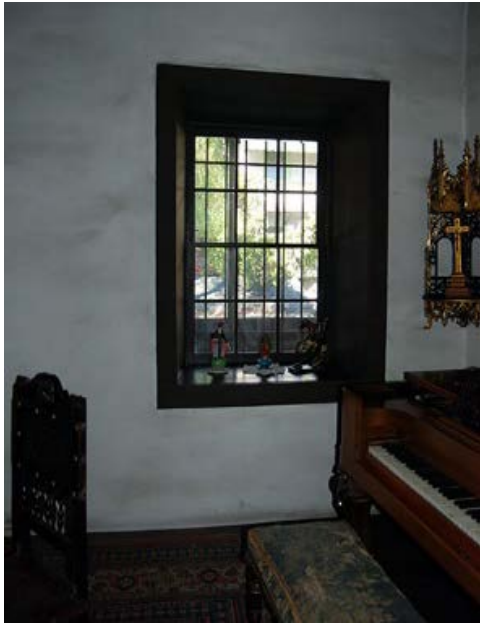
Figure 13: Window from interior.
