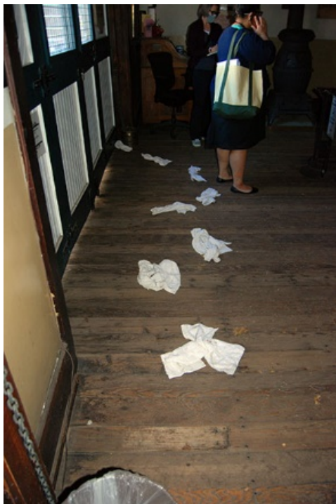
Figure 20: Threshold at apparatus door
