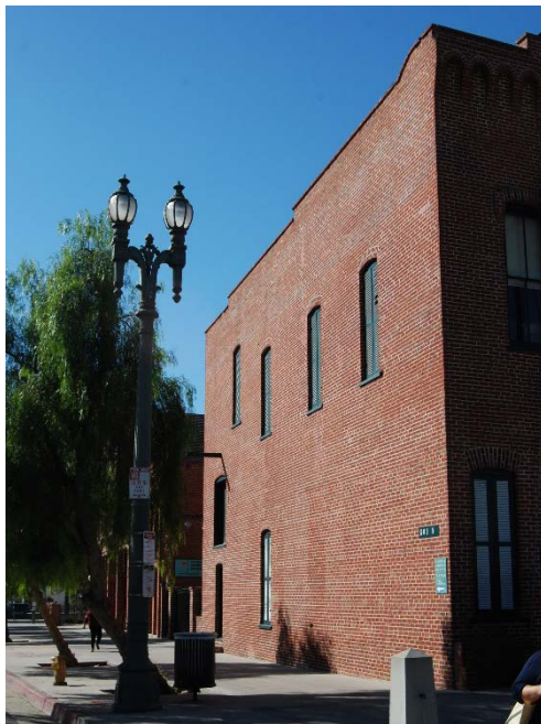
East façade of Plaza Firehouse; view to the southwest.
