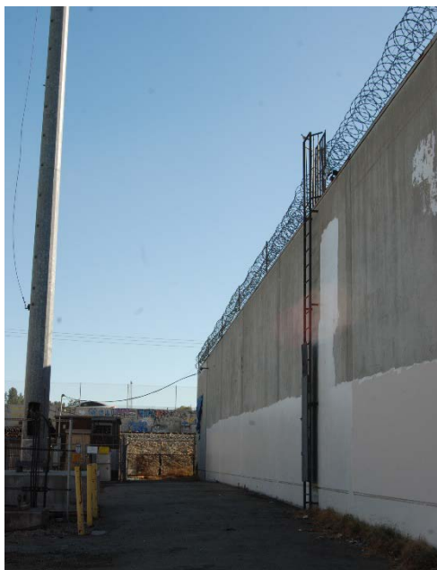
Figure 30: Exterior wall with barbed concertina wire.
