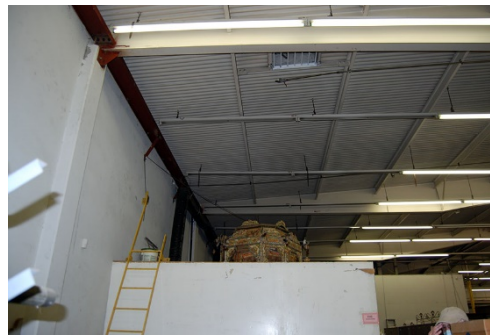
Figure 25: Interior surface of exterior concrete wall at connection to roof framing.
