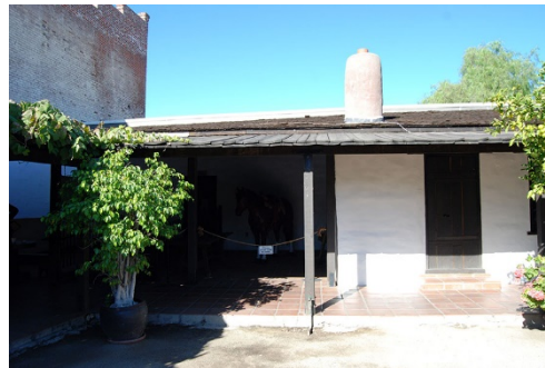
Figure 1: Wood shingle and plank roofing at east wall and corridor.
