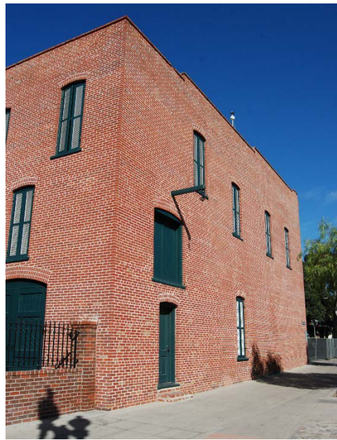
East façade of Plaza Firehouse; view to the northwest.
