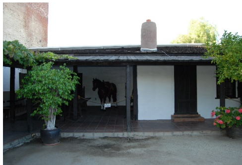
East façade of Avila Adobe; view to the northwest.
