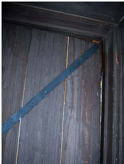
Figure 7: Daylight at exterior opening
