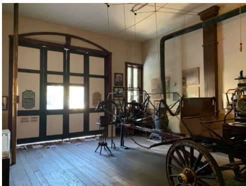
Figure 6: Overview of first floor of Firehouse facing north with strong light coming through barn door windows and side window. Also note gaps in doors and towels on floor.
