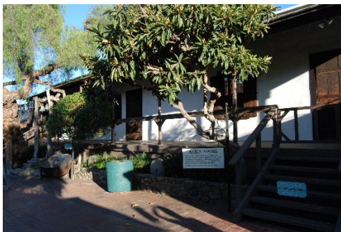
West façade of Avila Adobe; view to the east.
