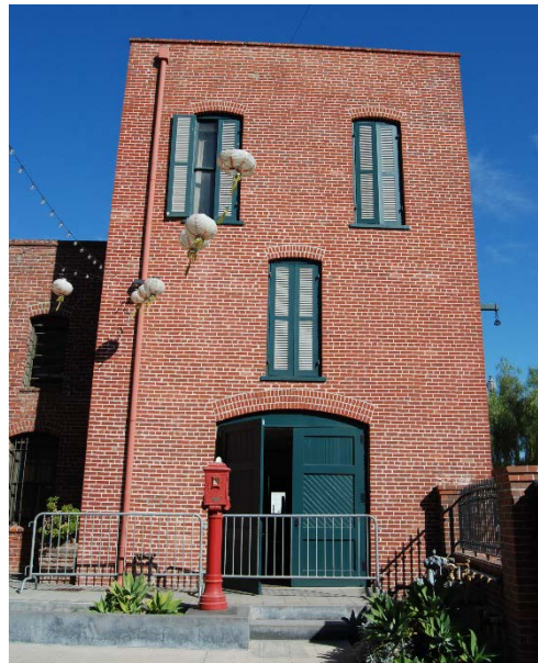
South façade; view to the north.
