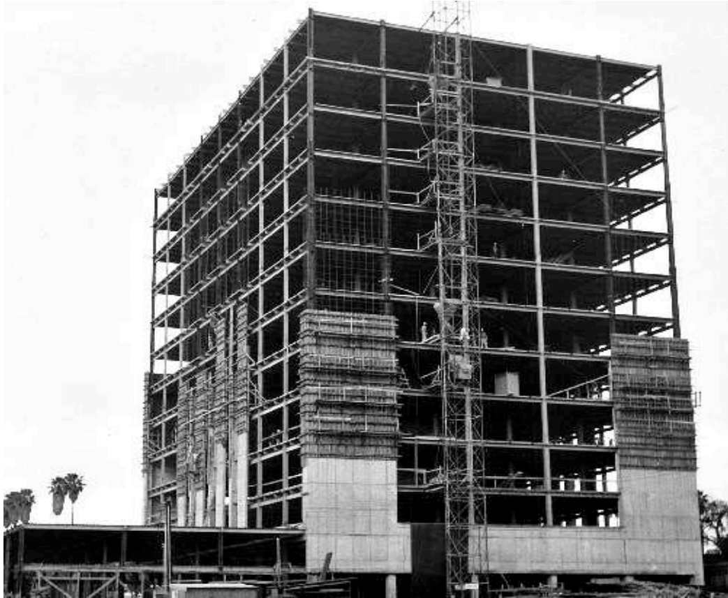
Figure 20. Triple Mariposa Building under Construction Showing Partial Concrete Sheathing and Areas Left for Curtain Wall. Brandow Archives.
