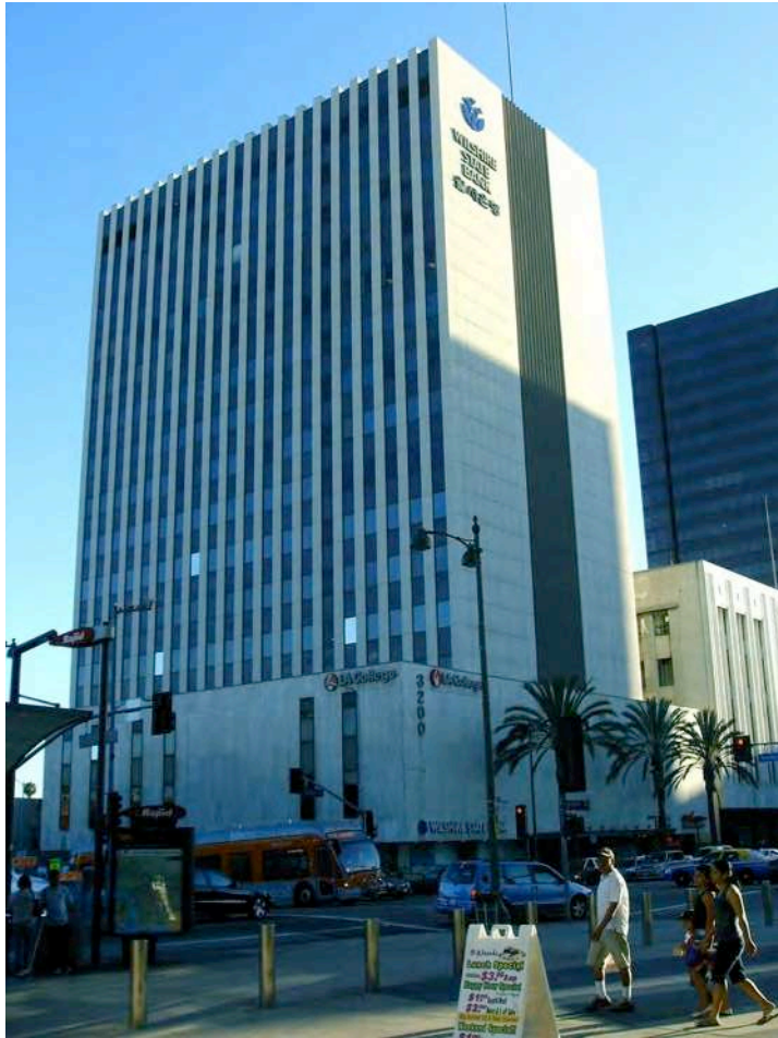
FIGURE 45. Pacific Indemnity Building (1962) Wilshire and Vermont Corner, 2009 Credle.
