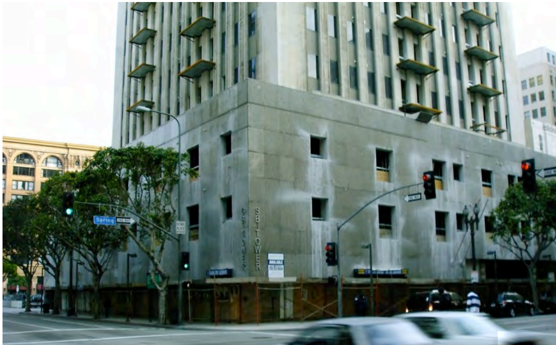
FIGURE 43. California Bank undergoing conversion in 2009 Credle.
