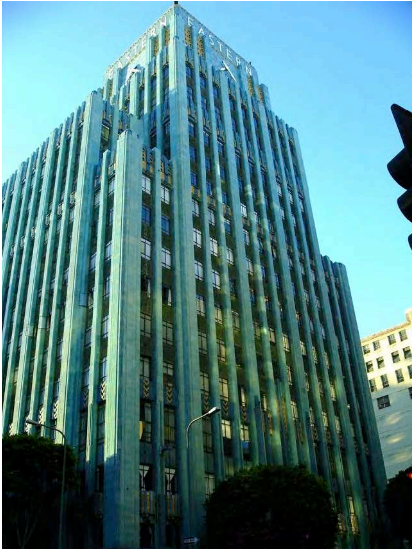
FIGURE 2. Eastern Columbia Building (1930) in 2009 Credle.
