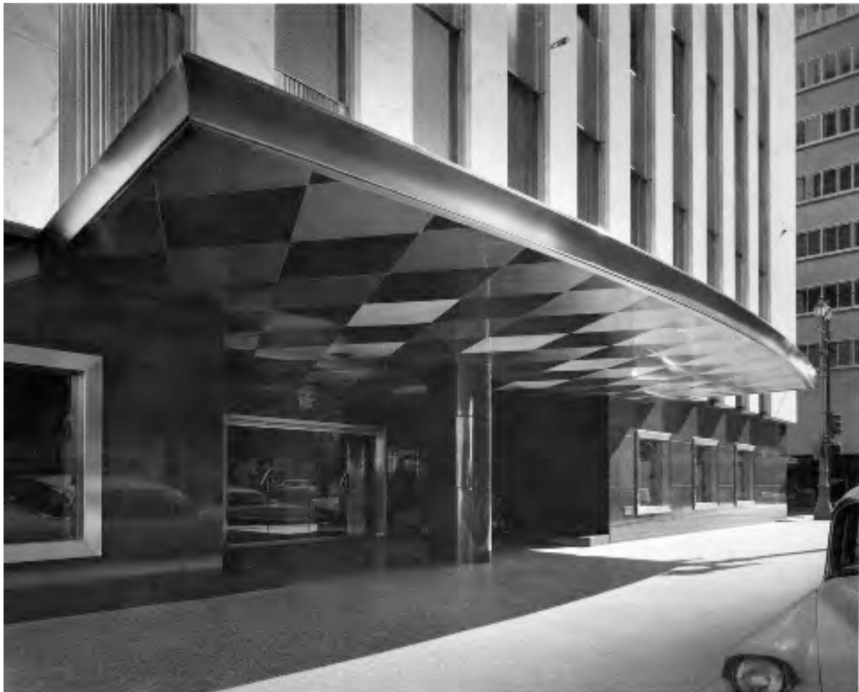
FIGURE 30. Superior/Standard 1954/55 Entrance showing Beelman's use of the stainless steel edged canopy. Getty Research Institute Julius Schulman Archive.
