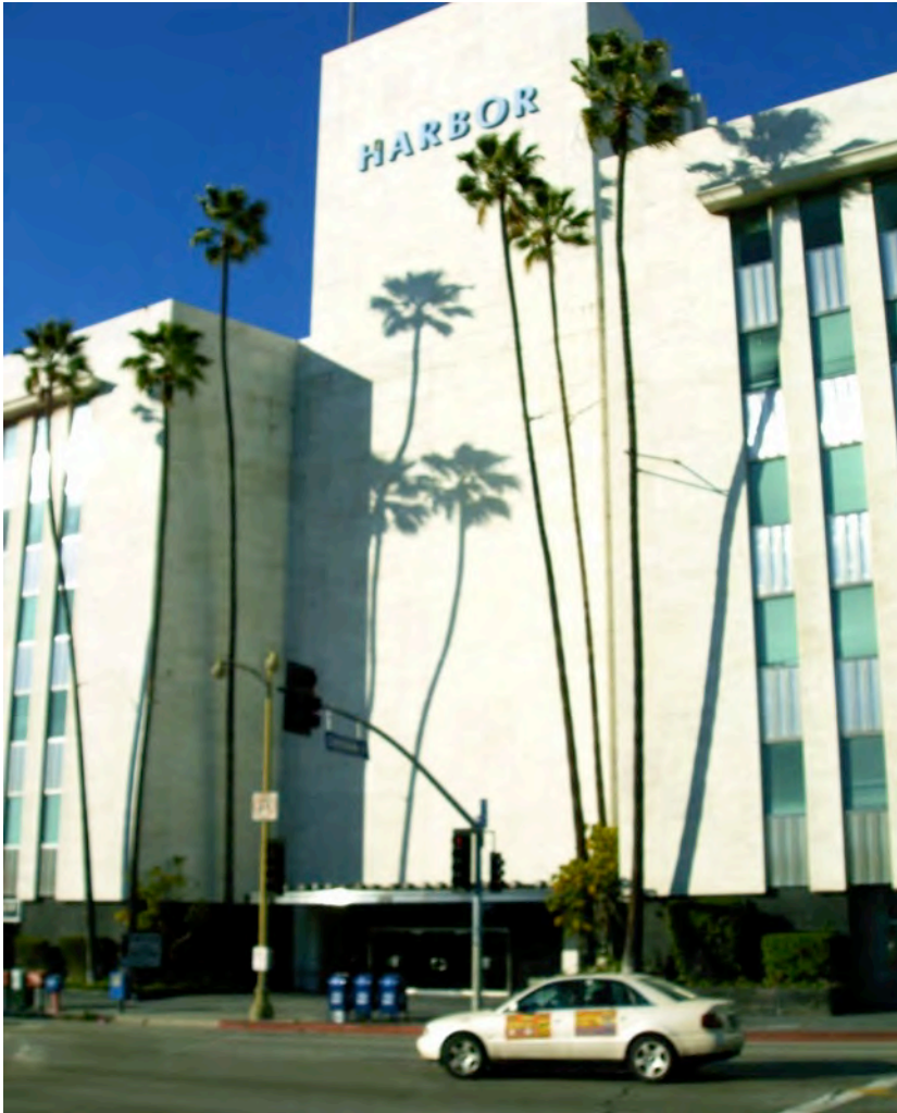
FIGURE 37. Tidewater Oil/Harbor Building (1958) Wilshire Boulevard Entrance in 2009 Credle.
