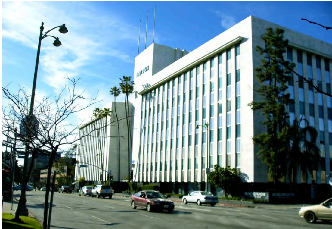
FIGURE 38. Tidewater Oil/Harbor Building Wilshire Boulevard Facade (1958) in 2009 Credle
