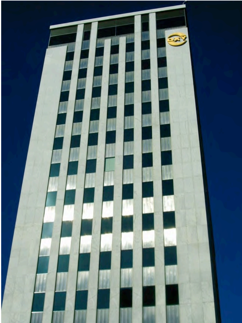
FIGURE 53. Kirkeby/Occidental Building (1962) West Façade Showing both the Scalloped Stainless Steel Spandrels and the White Marble Piers and Corners 2009 Credle.
