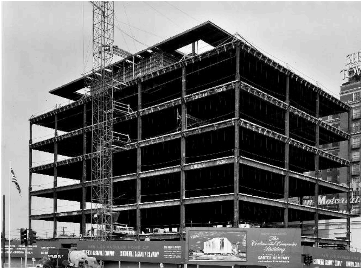
FIGURE 25. Continental Companies Building under Construction 1956 Brandow Archives.
