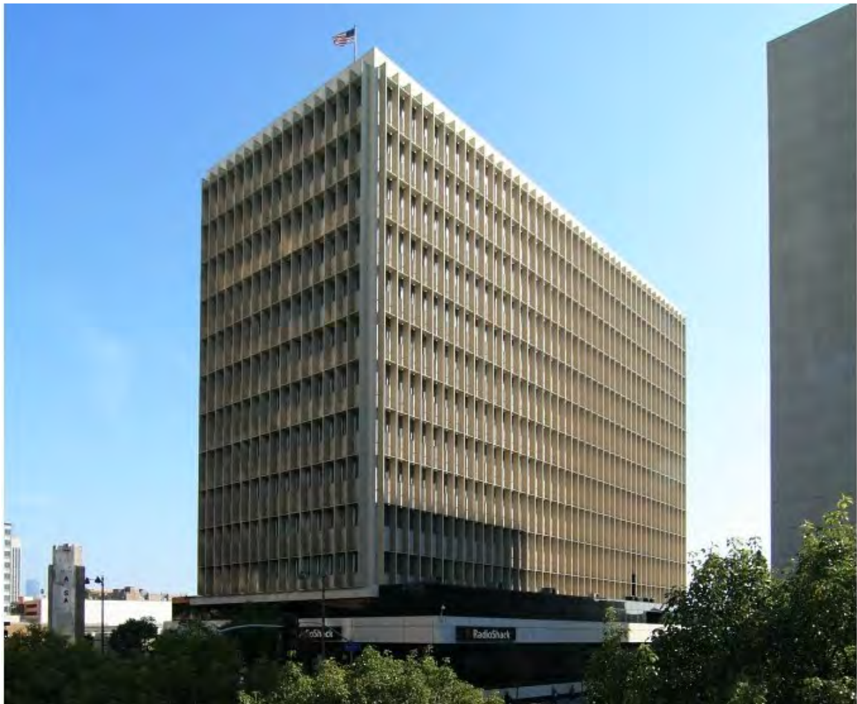
FIGURE 23. IBM Building 3424 Wilshire Boulevard at Mariposa Luckman and Pereira 1956-58 Photo Youarehere.com.
