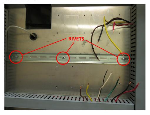
3. Drill out the heads of the three rivets to remove slotted mounting rail. Make a note of the various input and output wires.
