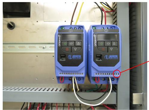
If terminals 10 & 11 have wires connected, remove and tie together. See step 9.
