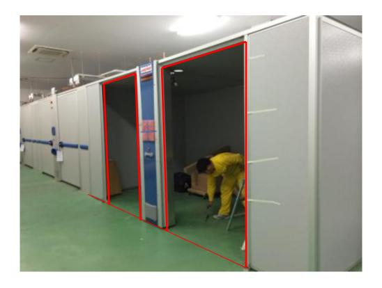
Line from front corner post extrusion left to right then install front panel, Adjust console position to same line with front panel
