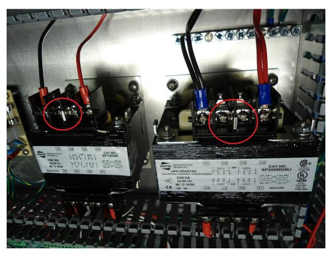
Following photo shows the jumper configuration for 380V supply (220V phase to Neutral) circled in red.
