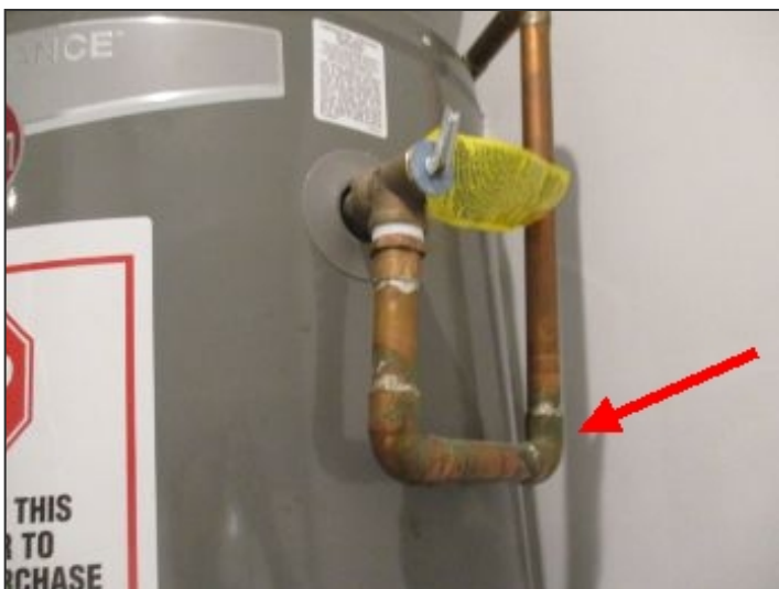
Missing drain valve at T&P drain pipe
