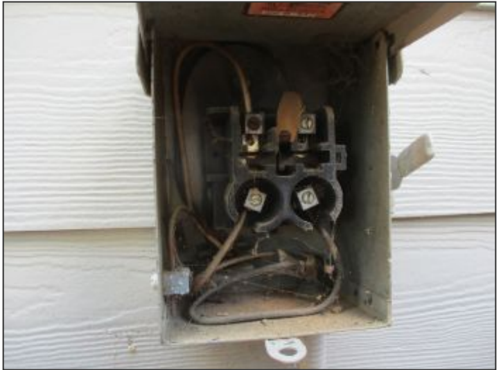
Missing deadfront cover at A/C disconnect
