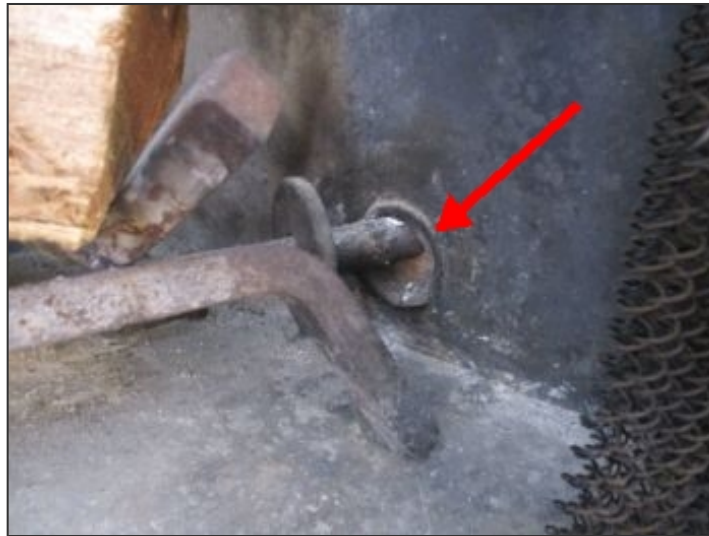
Opening at gas pipe in firebox
