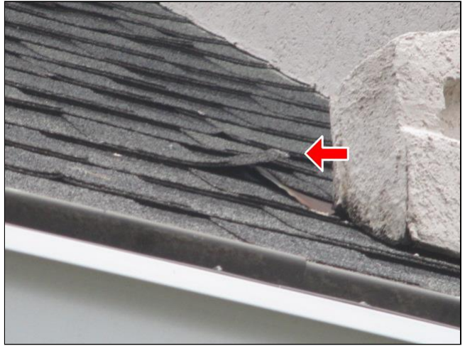
4.0 Item 17(Picture) Damaged shingle
