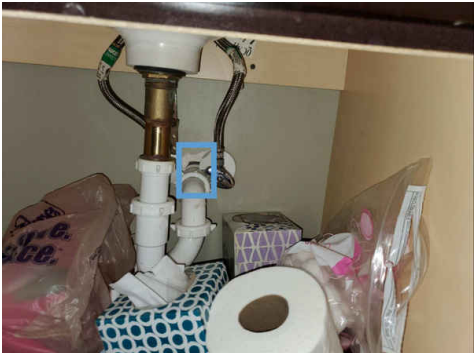
Foam Fill 1st Floor Bathroom
