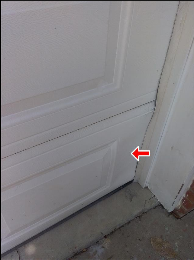
4.3 Item 1(Picture) Damage to garage door
