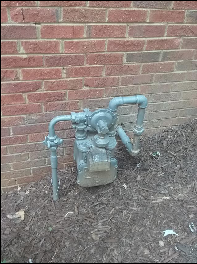
7.2 Item 1(Picture) External fuel service entry
