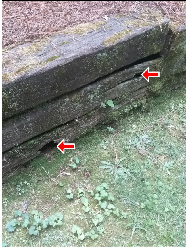
1.5 Item 2(Picture) Decay in retaining wall
