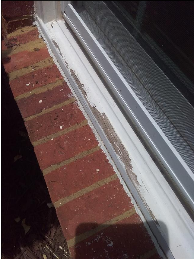
2.4 Item 1(Picture) Bare wood on window frame
