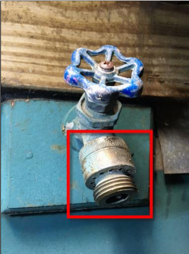
7.1 Item 2(Picture) Proper vacuum breaker installation
