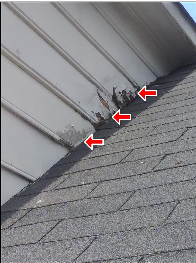
2.0 Item 1(Picture) Deterioration of siding
