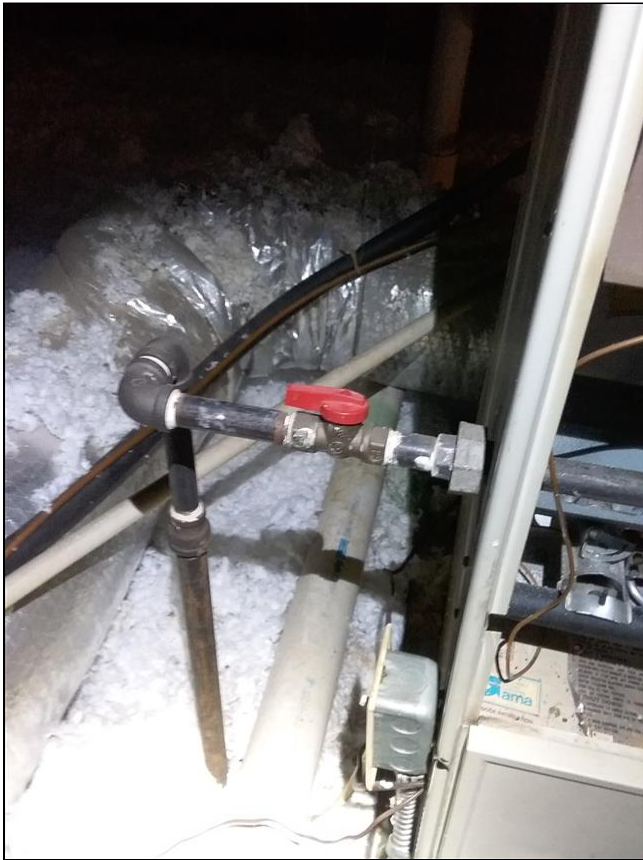
9.0 Item 4(Picture) No sediment trap installed
