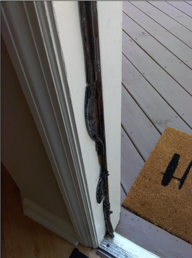
2.3 Item 1(Picture) Damaged weather stripping
