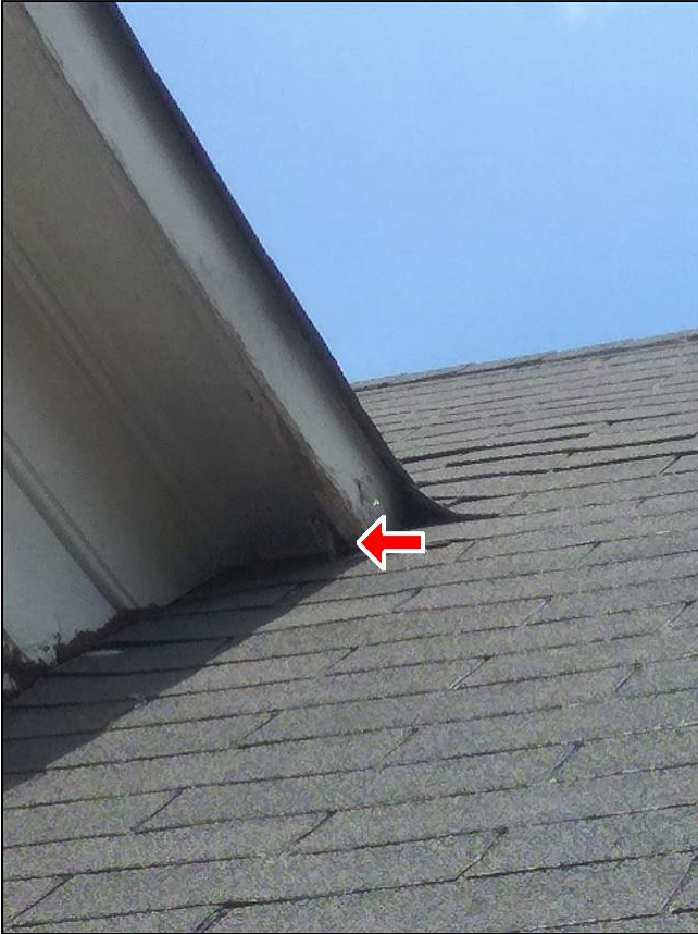
2.2 Item 1(Picture) Deteriorated fascia
