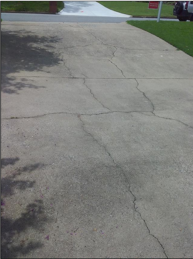
1.3 Item 1(Picture) Common cracks in driveway
