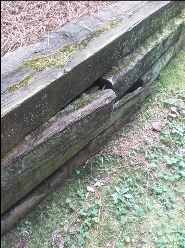
1.5 Item 1(Picture) Bowing retaining wall
