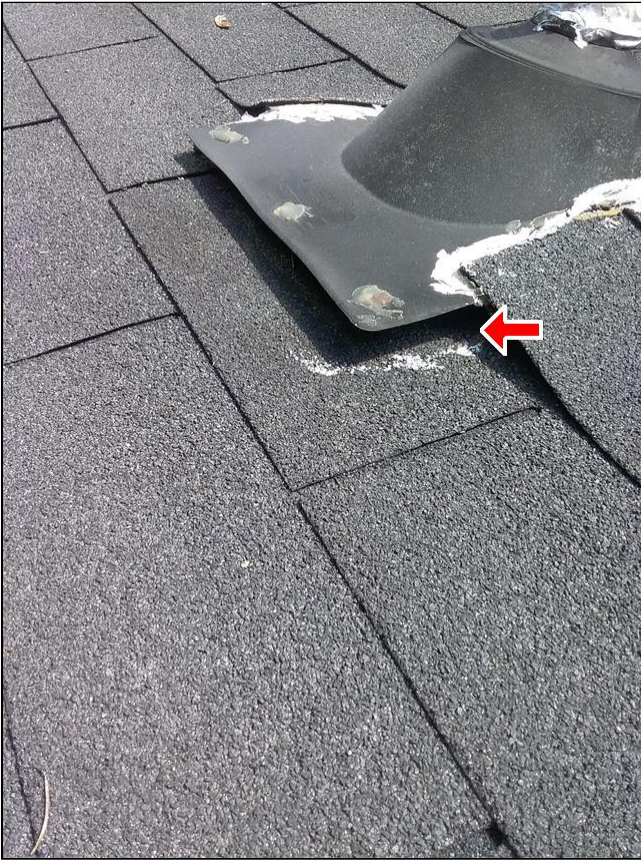
3.6 Item 1(Picture) Gap between flashing and roof
