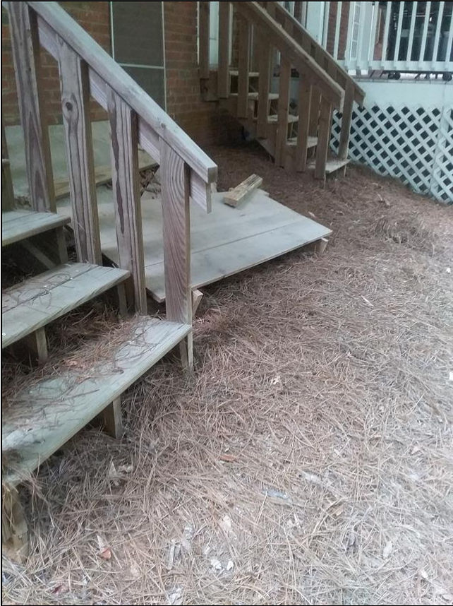
1.0 Item 2(Picture) No landing at exterior stairs
