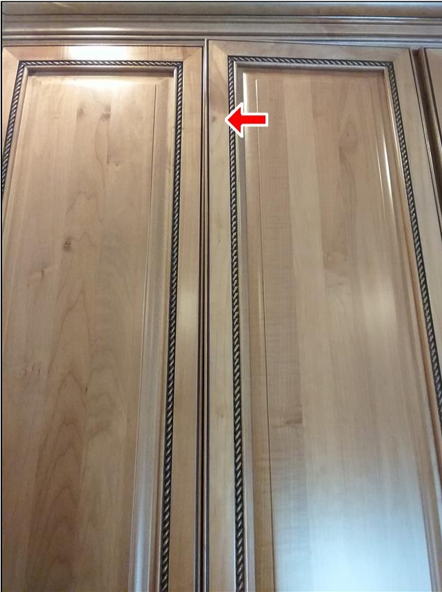
6.7 Item 1(Picture) Cabinet doors out of plumb
