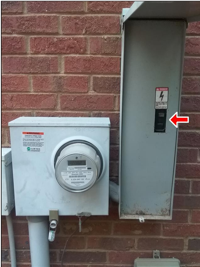
8.0 Item 1(Picture) External service and main disconnect
