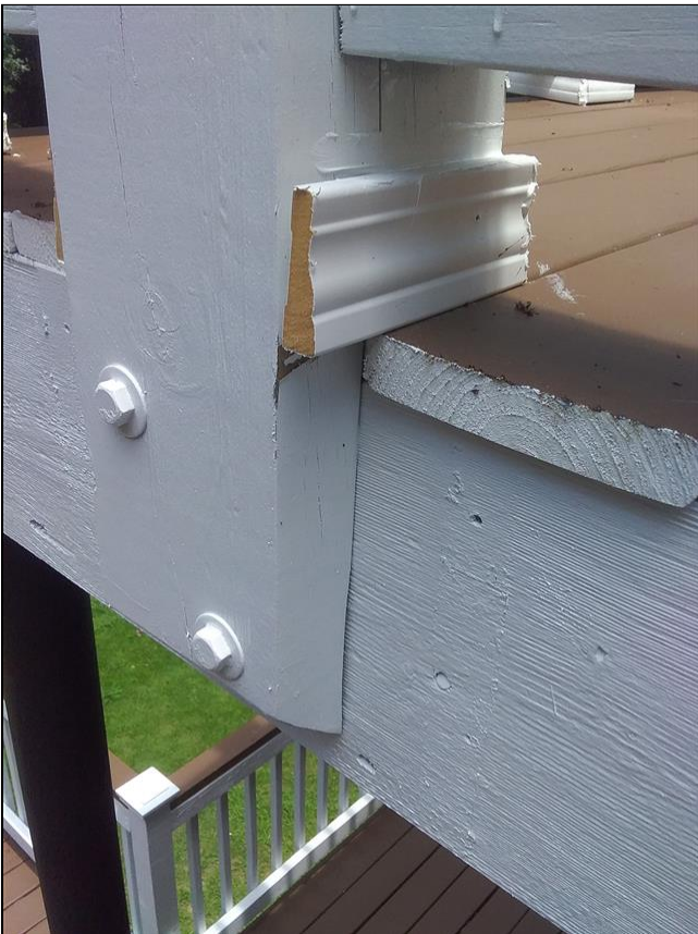
1.1 Item 1(Picture) Improper guard post attachment
