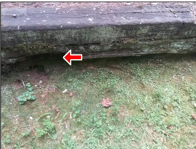
1.5 Item 3(Picture) Decay in retaining wall
