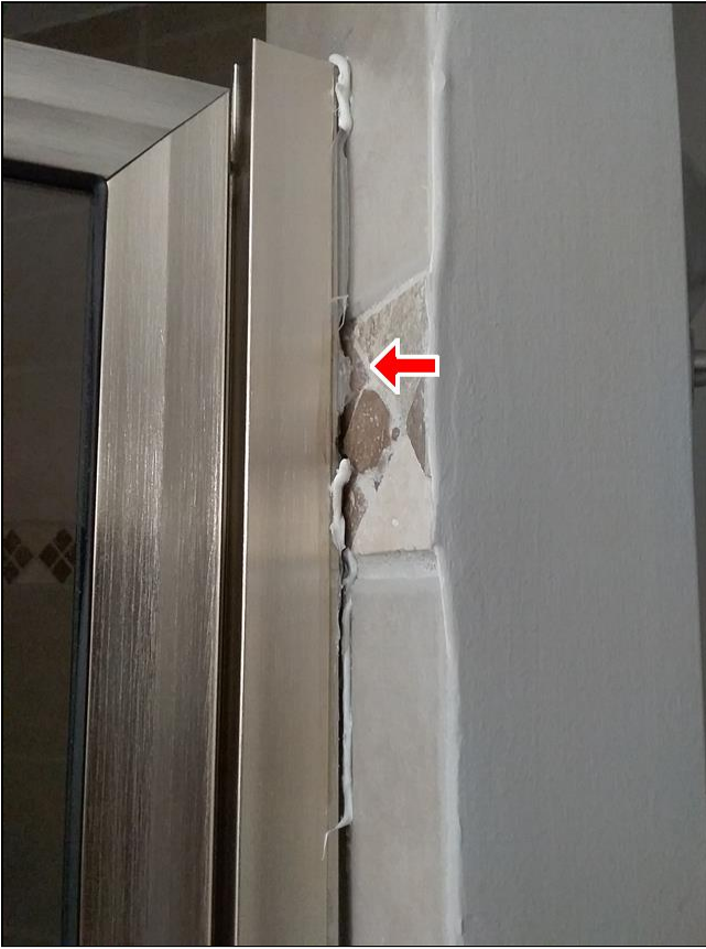
7.5 Item 4(Picture) Shower door loose at hinge
