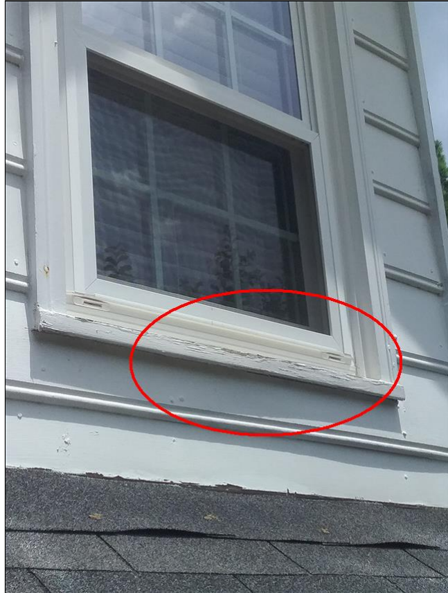
2.4 Item 2(Picture) Bare wood on window frame
