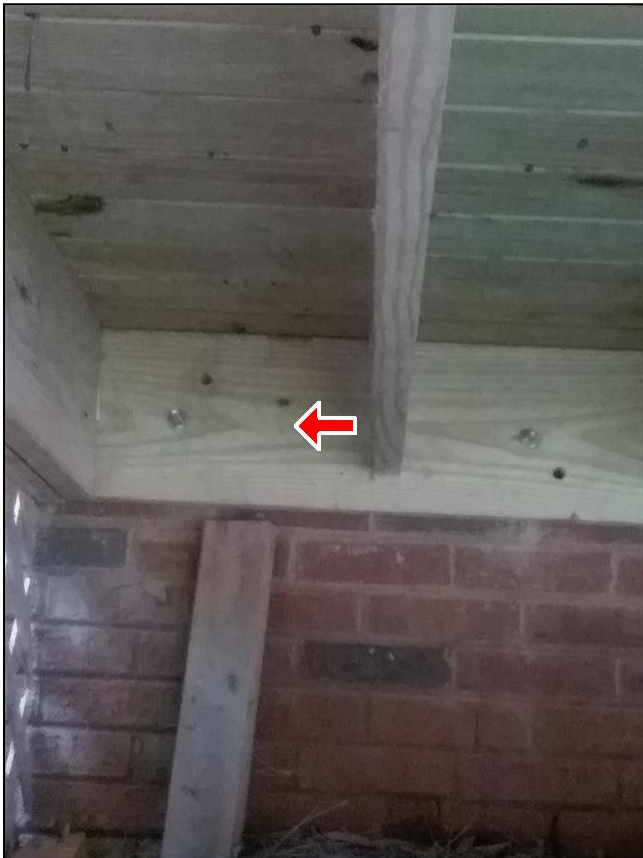
1.1 Item 6(Picture) Insufficient attachment
