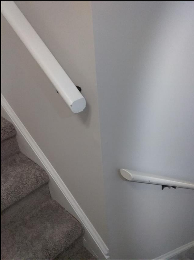
5.3 Item 1(Picture) Non continuous hand rail
