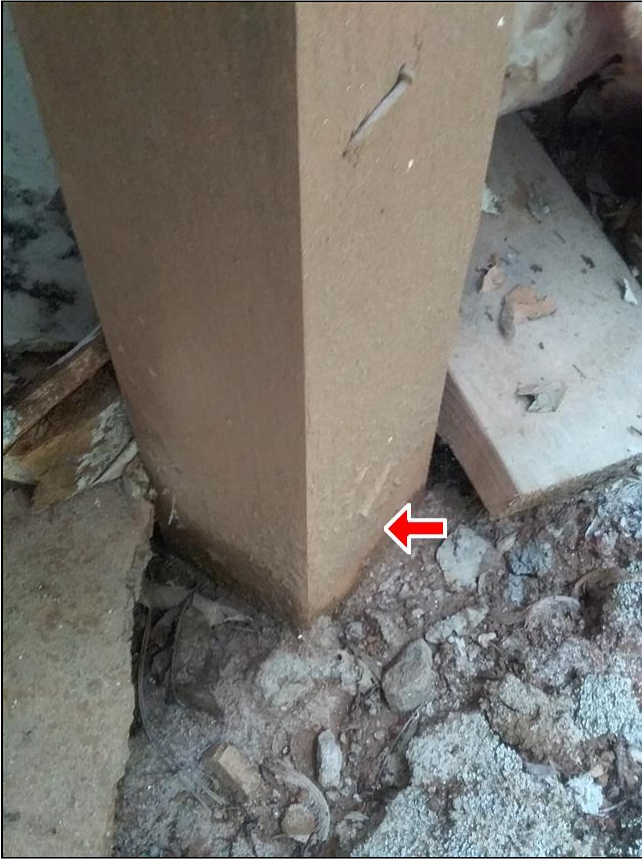
1.1 Item 11(Picture) Post in ground contact
