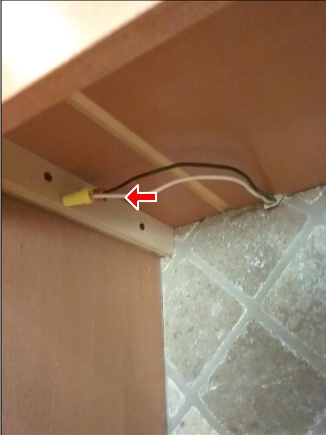
8.2 Item 1(Picture) Exposed wiring
