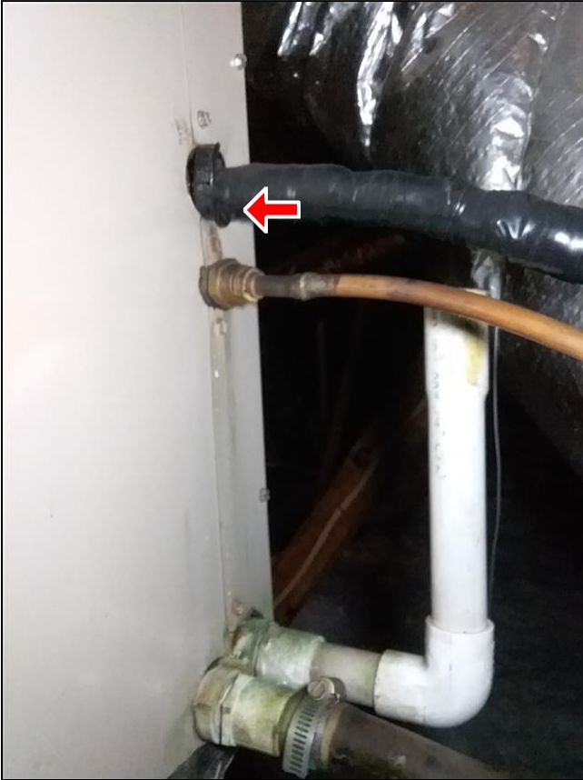
9.0 Item 6(Picture) Leak noted at rear of furnace
