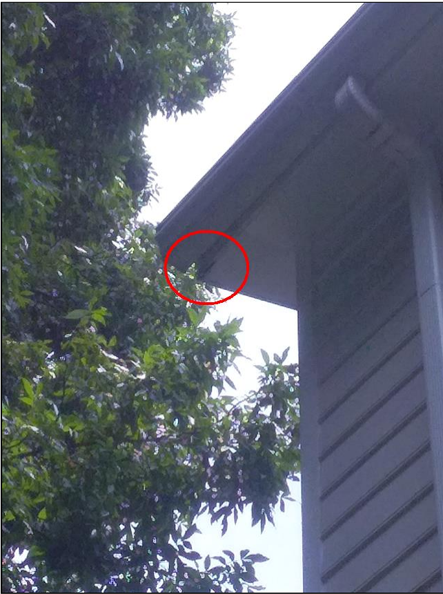
2.2 Item 2(Picture) Deteriorated fascia
