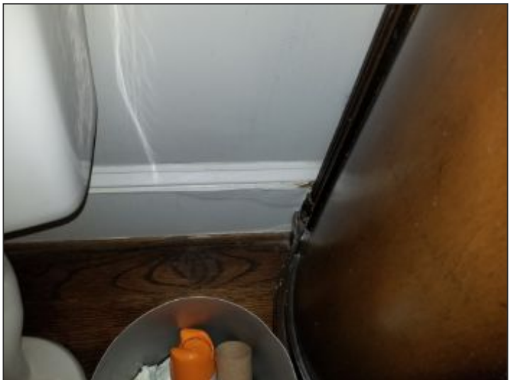
Evidence of a leak at half bathroom
