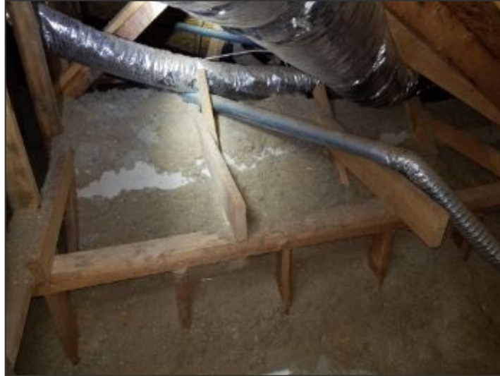
Missing insulation above master bathroom
