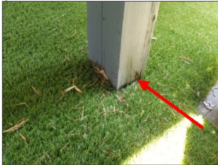
Post rot at deck stair landing
