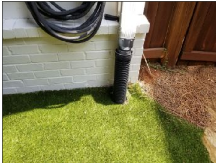
Underground downspouts present for improved drainage
