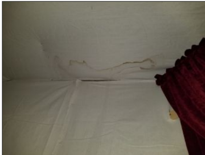
Evidence of a leak below kitchen sink - water stain on basement ceiling below
