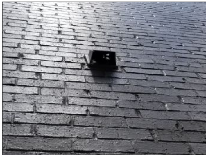
Damaged fresh air vent cover
