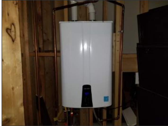
Tankless water heater located in basement
