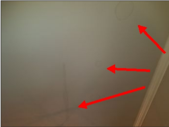
Water stains at eat in kitchen ceiling
