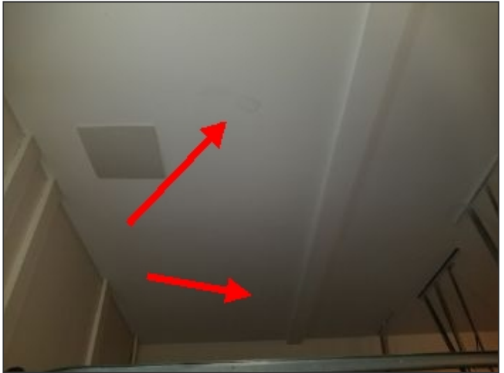
Water stains at garage ceiling
