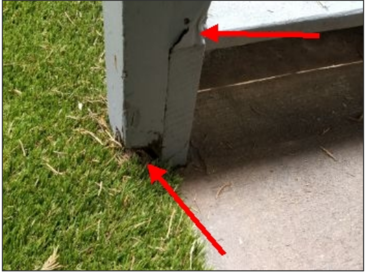
Damaged wood at rear deck stair rail posts
