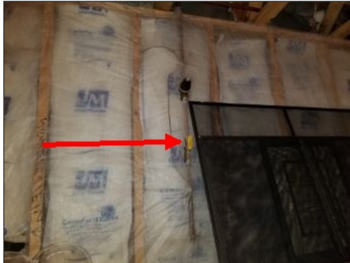
Main water cut-off handle located in basement
