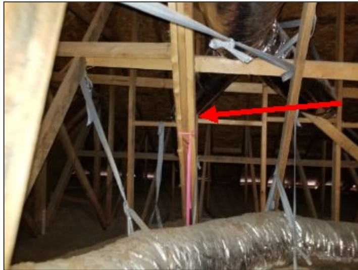
Adequately repaired roof truss in attic near pull down ladder
