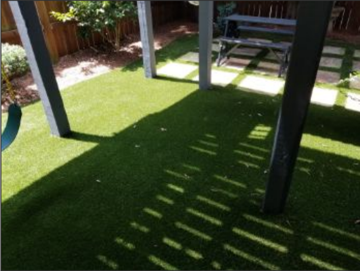
Wood posts below grade at rear deck
