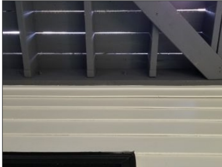
Good flashing and bolting at rear deck
