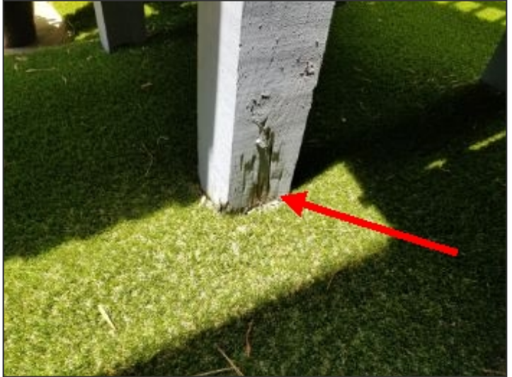
Post rot at deck stair landing
