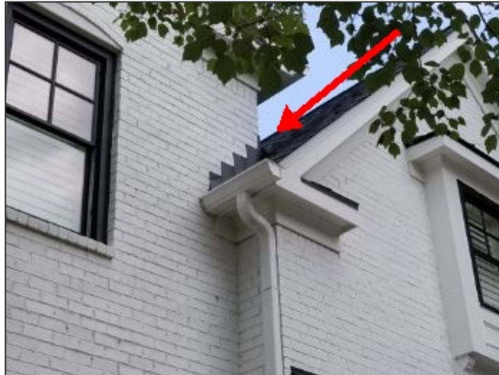
Good flashing practices at intersecting walls
