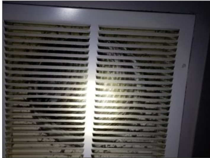
Dirty ducts - view of second floor return vent
