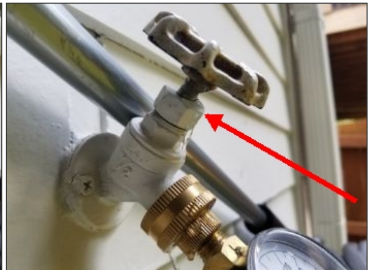
Active leak at rear hose bib handle
