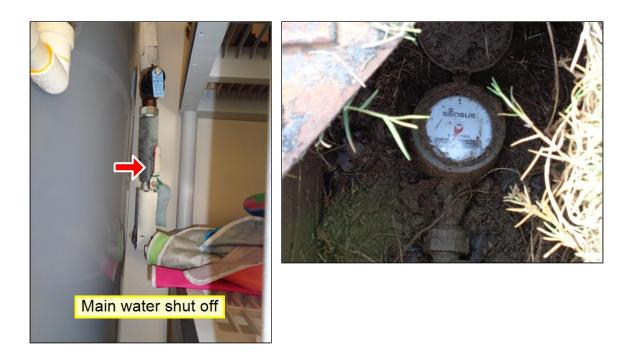
SERVICE / REPAIR: The water pressure tested at over 80 PSI. This is considered excessive and adjustment of the pressure regulator is necessary. Correct to have between 40 and 80 PSI. Item 3(Picture)
