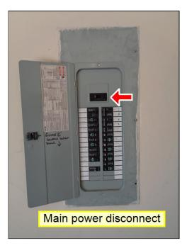
SAFETY / HEALTH: The screws currently being used to attach the panel cover are improper. These screws have pointed ends and can pierce the insulation of the wires leading to a short circuit or electrical fire. Only blunt ended screws should be used. Item 2(Picture)
