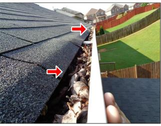
SERVICE / REPAIR: Improper slope of the gutters observed located at rear patio. The gutters should be sloped so that all water will drain toward a downspout. Have a roofer or gutter installer evaluate and repair or replace to the extent found. Item 7(Picture) Item 8(Picture)
