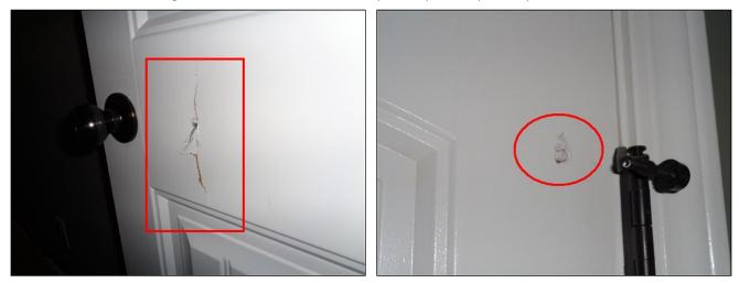
GENERAL NOTE: Door stops are typically installed to provide protection to walls from door knob contact and generally found in wall, floor or hinge mount types. Some found either damaged or missing and consider having installed.Item 5(Picture) Item 6(Picture) Item 7(Picture) Item 8(Picture)
