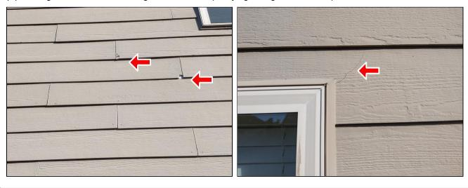
(4) Wood trim and siding and direct contact with soil. Is required to be a 2 to 4-in gap between siding/trim and soil. This is to prevent water damage and/or wood boring insect damage.
