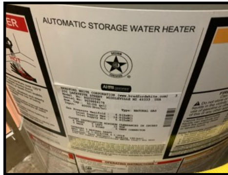
Bradford White 50 gal nat gas water heater, 2017 model
