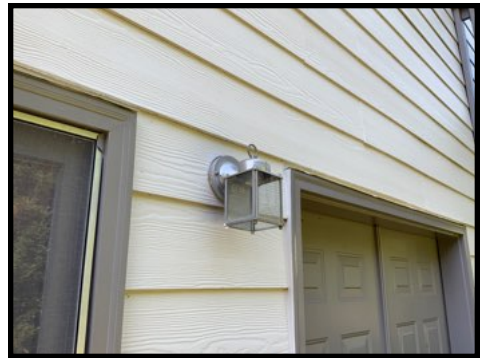
Inoperable light fixture at the rear basement door
