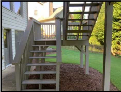
Open risers at exterior stairs
