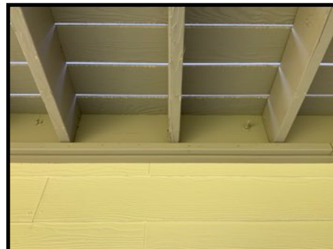
Deck appears to be properly secured and flashed
