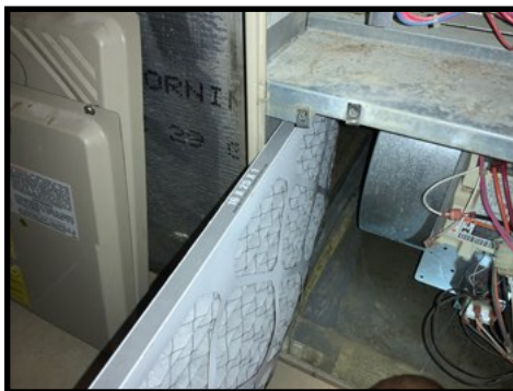
16x25x1 filter installed at the main level furnace
