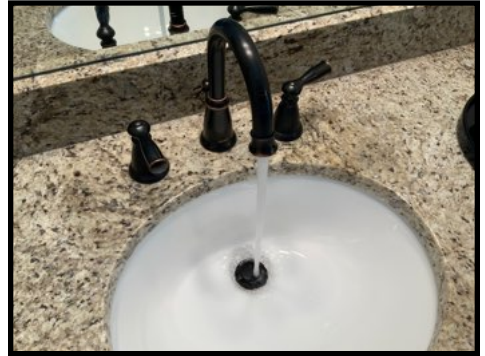
Non functioning drain stopper at the left side master bathroom sink
