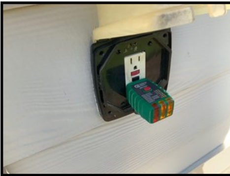
Faulty GFCI outlet at the right side of the home
