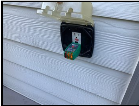
Faulty GFCI outlet at the rear deck
