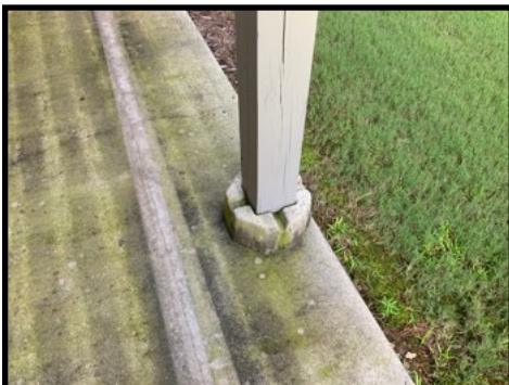
Pre-cast footings should be replaced with adequate/secured footings
