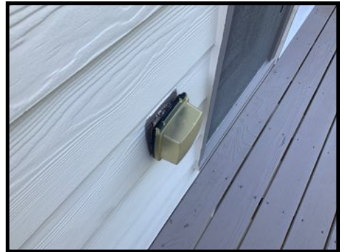
Loose cover at the rear deck
