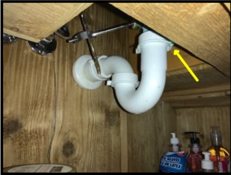
Active leak at the basement bathroom sink drain
