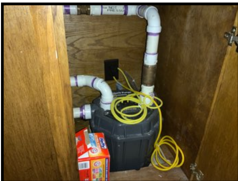
Mini ejector pump located in the wet bar
