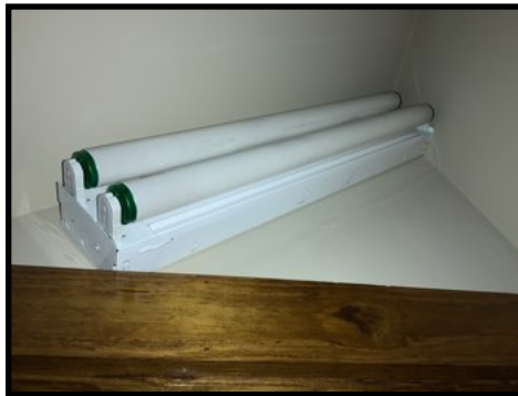
Inoperable light fixture in the basement bedroom closet
