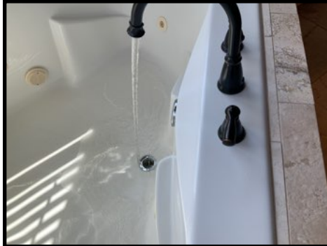
Missing drain stopper at the master bathroom tub
