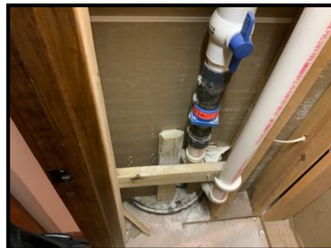
Ejector pump located in the basement
