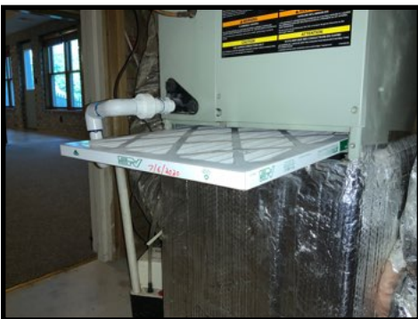
16x20x1 filter installed at the basement level furnace
