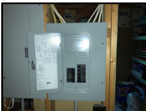
GE sub panel located in the basement
