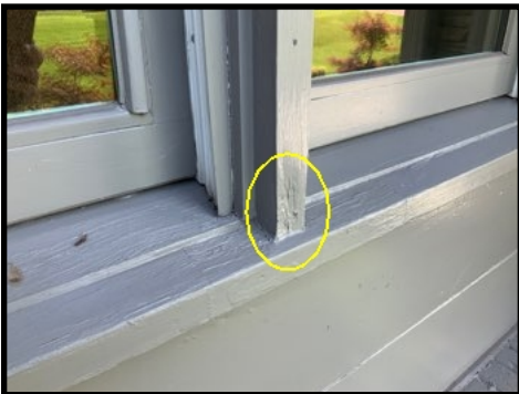
Damaged trim at the front sitting room window
