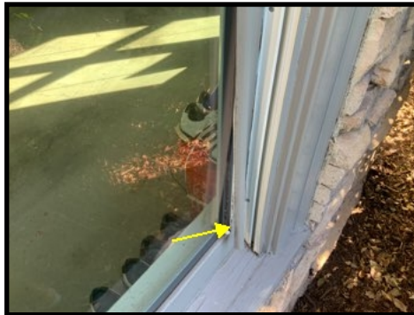
Damaged trim at the front garage window
