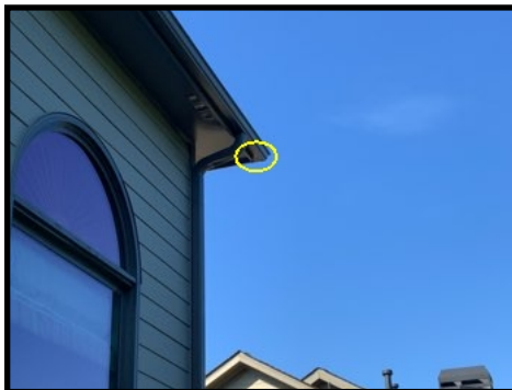
Damaged fascia at the left rear corner of the home
