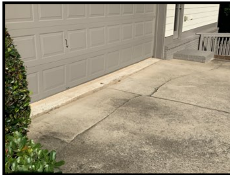
Cracked/displaced section of driveway
