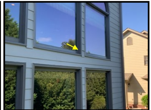
Damaged trim at the rear living room window
