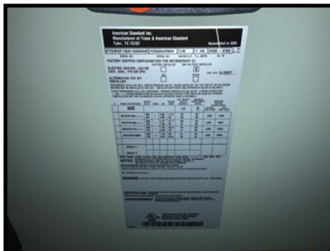
Trane electric furnace, 2007 model
