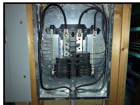
Interior wiring in the sub panel
