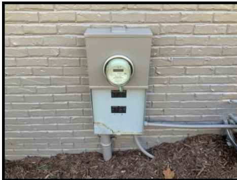
Electric meter and 200 amp shut off located at the left side of the home
