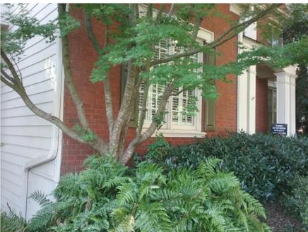
**28:** Trees are touching or overhanging the front right and rear center of the roof. Recommend trimming to avoid roof surface damage and wildlife entry.
