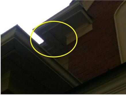
**39:** Unsealed caulking gaps observed at penetrations for wires/pipes/vents and dissimilar material junctions including and not limited to the front right trim, right side gas pipe, rear right window, rear center window, exterior lighting fixtures and electrical outlets . All penetrations should be completely sealed to prevent any possibility of water entry. Failure to properly seal all gaps can result in moisture damage to the framing.
