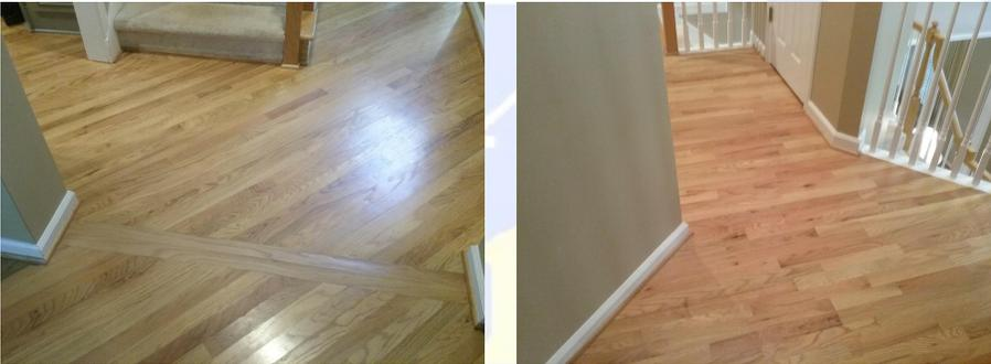
**147:** Squeaks are the result of two materials rubbing against each other. Repairs involve securing the floor so that it does not move. Unfortunately, due to the normal expansion and contraction of the building it is not possible to stop all the squeaks everywhere. You can usually stop one or at least move it from a given area, by screwing or nailing the floor in the area that is making the noise.
