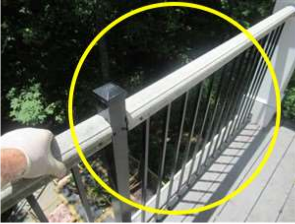
Photo 6-1 Master bedroom deck railing.
