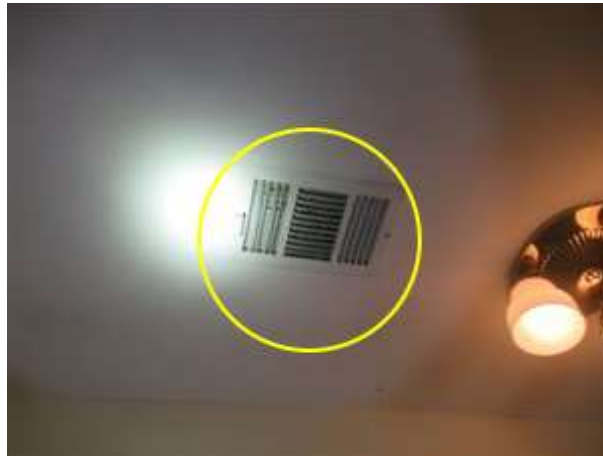
Photo 39-2 Upstairs hallway by the laundry room.
