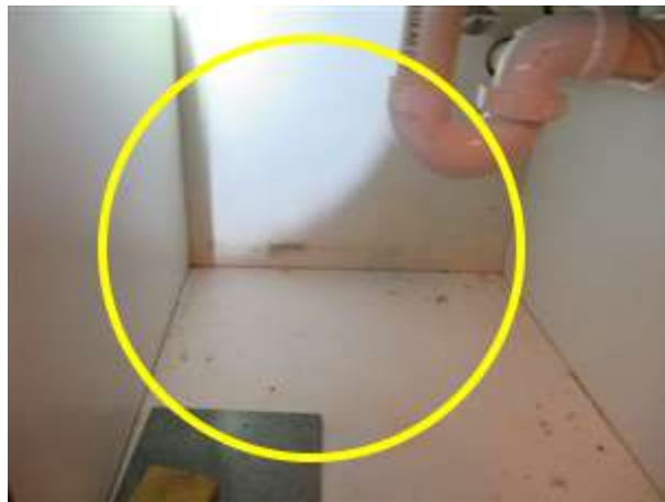
Photo 94-4 Basement bar sink cabinet.
