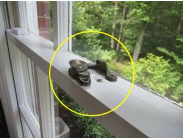
Photo 87-1 Front office window.
