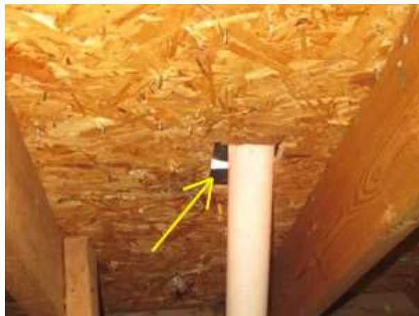
Photo 22-2 View from inside the attic.
