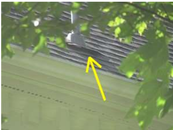
Photo 22-1 Located on the right side of the roof.
