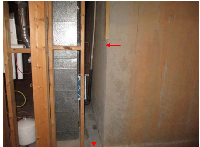
A qualified contractor should re-install the wall stud and sill plate along the foundation behind the main floor furnace in the basement.
