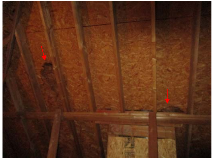
Moisture stains were present on the roof decking above the chimney chase in the back, left corner of the upper attic.
