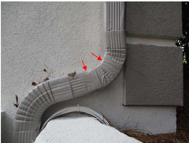
The lower portion of the downspout has been taped above retaining wall at the left, front corner of the home due to this section of the downspout being rusted.
