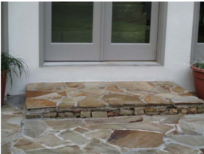
The excessive height between the threshold and the stone step outside the exterior French doors in the rear wall of the family room presents a possible trip hazard.
