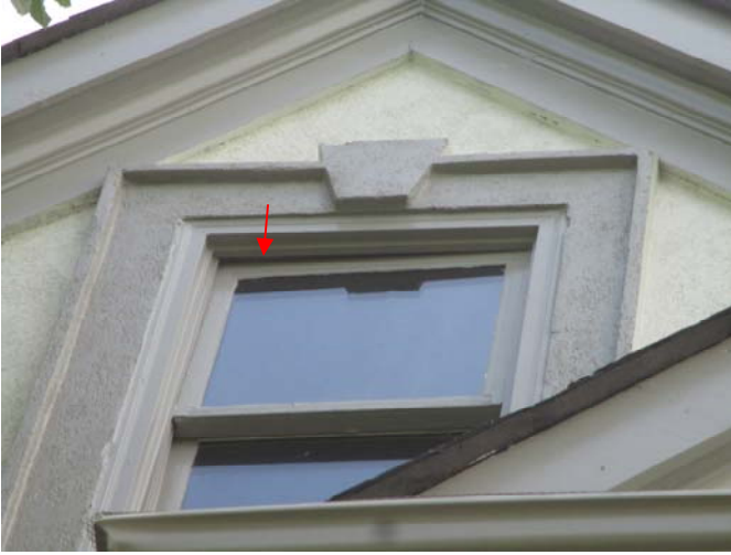
The upper sash is displaced in the window located in the front wall of the attic.
