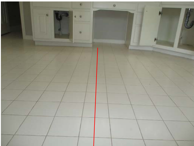
A ridge was present in the center portion of the tiled floor in the master bathroom which has caused a hairline crack in the floor tiles.
