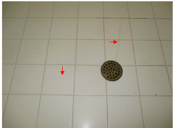
Hairline cracks were present in the tiles around the drain in the floor of the master shower stall, which is mainly cosmetic in nature.
