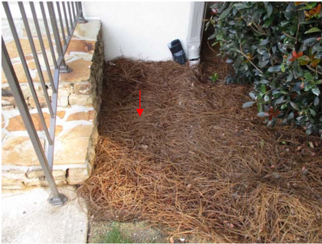
A basin was present in the soil on the right side of the stone steps outside the exterior door in the laundry room.
