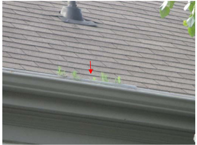
The insides of the gutters and downspouts should be cleaned prior to closing as part of routine maintenance.
