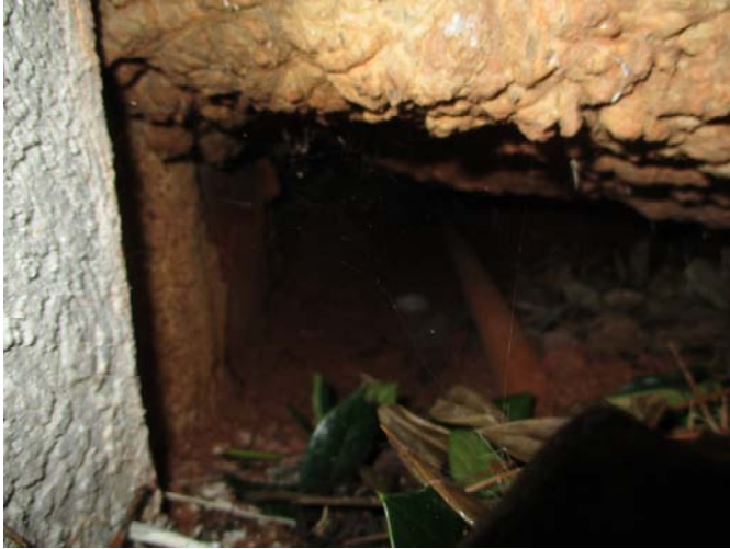
A large void was present in the soil below the rear portion of the front stoop.
