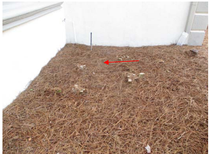
Negative grading was present in the soil outside the front wall of the formal dining room.
