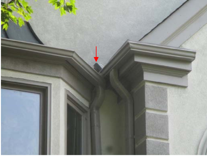
Raintek kick-out flashing has been installed in the stucco system at the primary roof termination located above the right side of the bay window cavity in the left, front bedroom.
