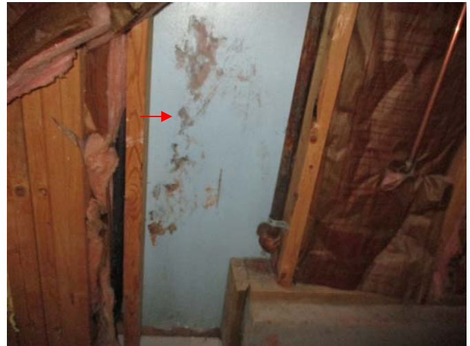
There appears to be past termite trails on the rigid foam wall sheathing located above the lower step-down in the foundation in the back, left corner of the basement.
