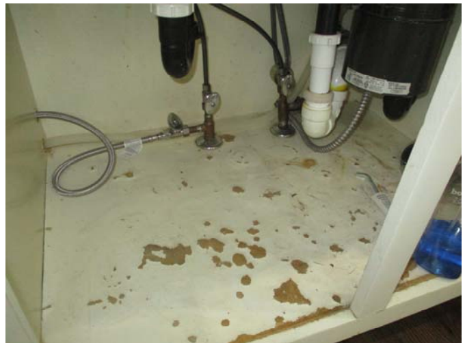
Moisture damage was present on the cabinet shelving below the kitchen sink.
