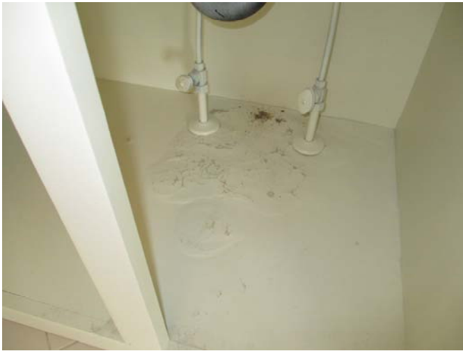
Moisture damage was present on the cabinet shelving below the right sink in the master bathroom.
