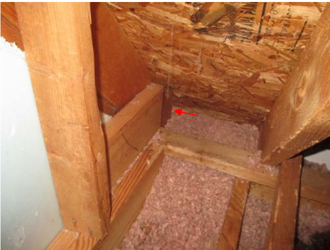
A rodent access hole was present above the gable return in the left, front corner of the upper attic.
