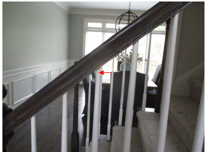
Replace the cracked spindle in the railing on the right side of the stairwell located in the right, front corner of the family room.
