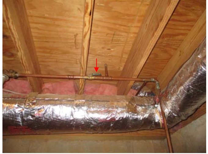
The shut-off valve on the main waterline is located at the right, front corner of the basement ceiling (below the formal dining room).
