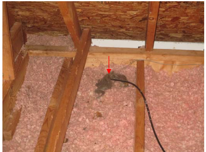
A squirrel carcass was also present in the insulation in the left, front corner of the upper attic.
