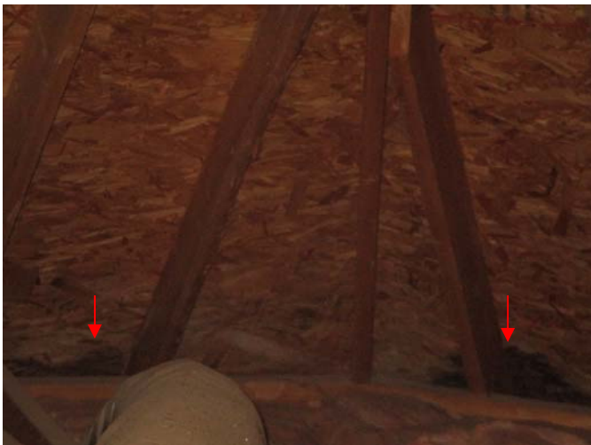
Moisture stains were present on the roof decking above the bay windows in the rear wall of the master bedroom.
