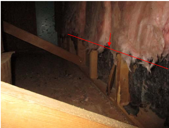
A qualified contractor should replace the rodent damaged batt insulation in the left wall of the knee wall portion of the attic located off the right wall of the master bedroom closet.
