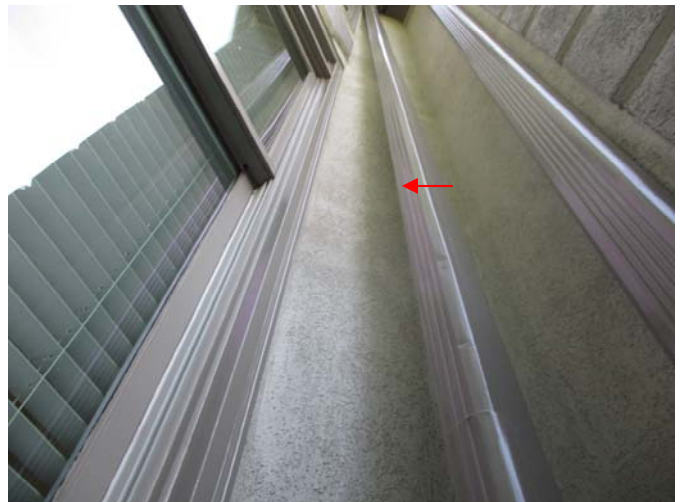
A qualified contractor should secure the downspout to the EIFS system on the right side of the bay windows at the left, front corner of the home and ensure the downspout straps penetrating the EIFS system are sealed with caulking.
