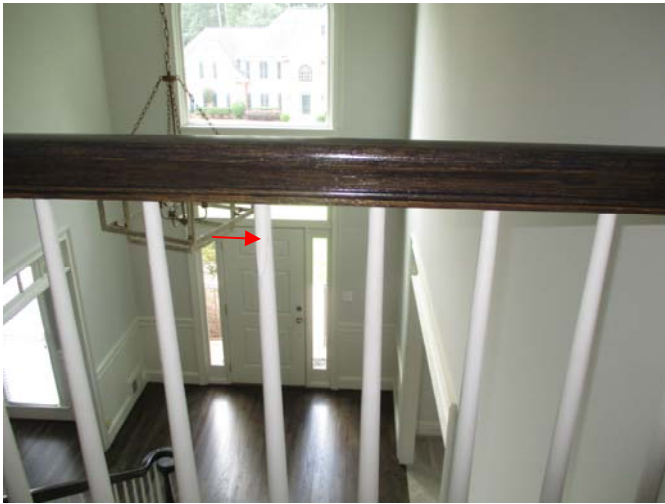
Replace the cracked spindle in the railing at the top of the stairwell in the foyer.
