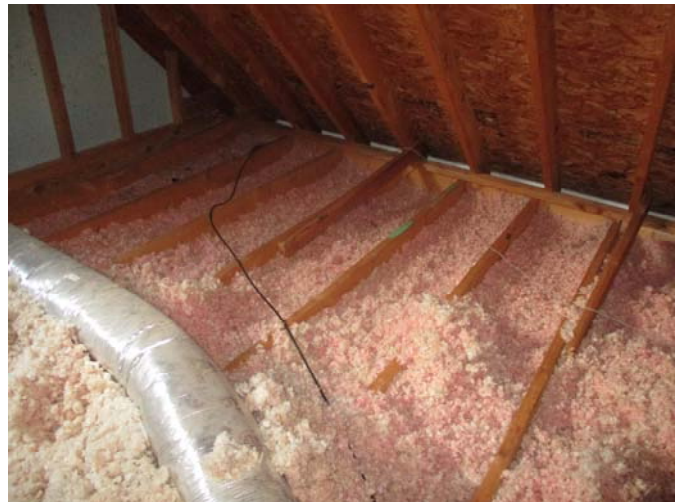
The blown-in insulation in the floor of the upper attic has been trampled in various areas from previous rodent activity.
