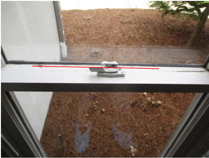
Minor moisture damage was present on the interior frame below the upper piece of glass in the right window in the formal dining room.
