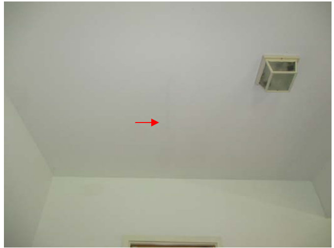
There appears to be inactive moisture stains on the rear portion of the garage ceiling.
