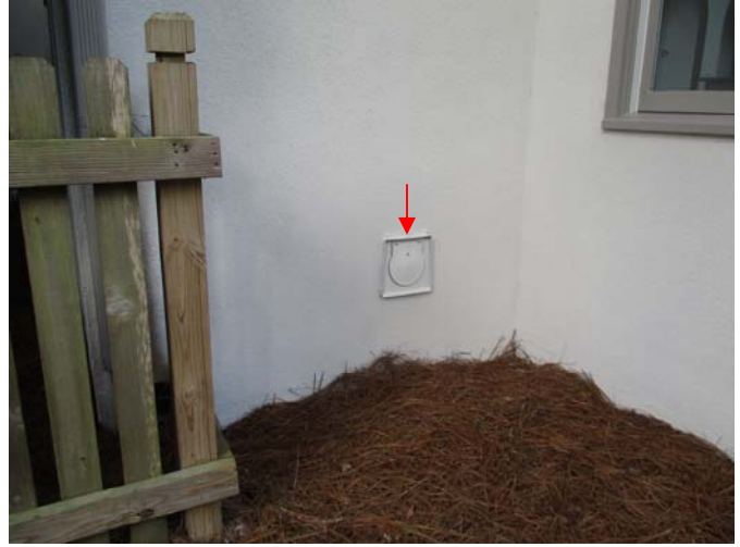
A qualified contractor should install the missing venthood over the vent for the downdraft exhaust fan located below the rear wall of the kitchen.
