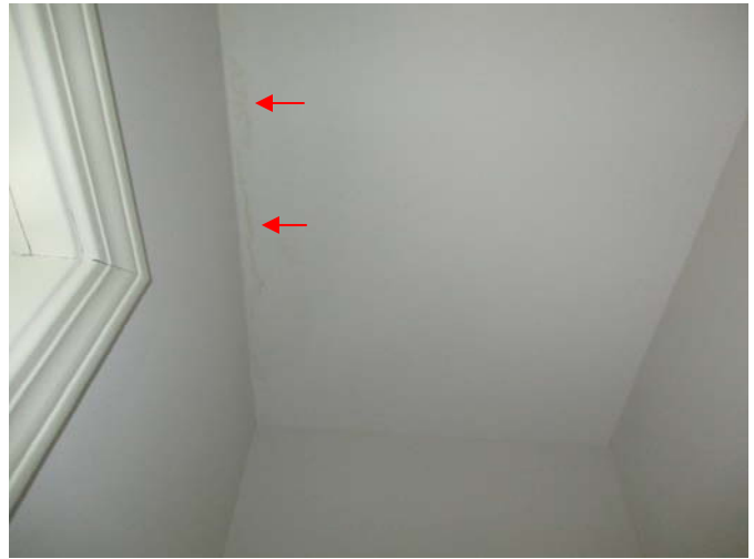
Inactive moisture stains were present on the ceiling of the rear closet in the back, left bedroom, which may be related to gutter overflow.
