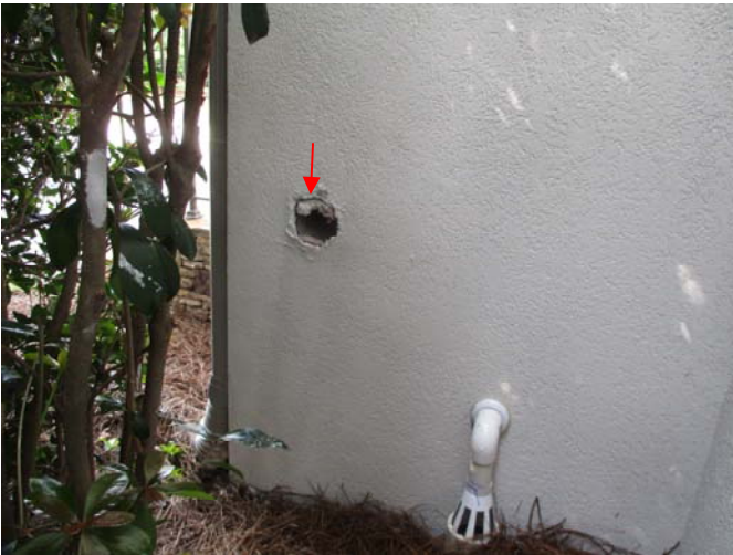
A qualified contractor should install the missing venthood over the dryer vent located outside the rear wall of the laundry room.
