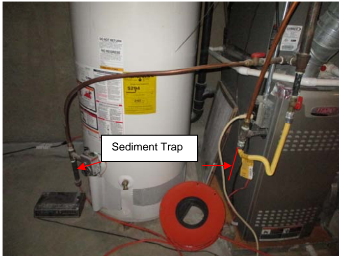
A sediment trap is missing on the gas line entering the main floor furnace.
