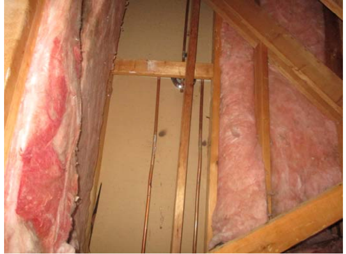
A qualified contractor should install the missing insulation in the rear wall of the knee wall portion of the attic located off the right wall of the master bedroom closet.
