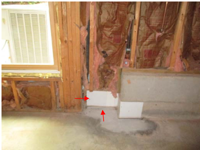
A qualified contractor should re-install the wall studs and sill plate along the lower step-down in the foundation in the back, left corner of the basement.
