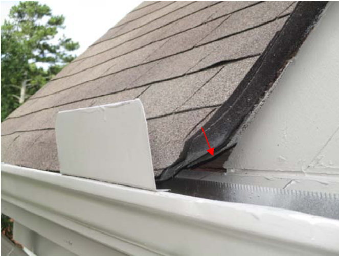
A construction gap was present between the fascia board and the roof decking at the bottom of the roof valley located above the garage door.
