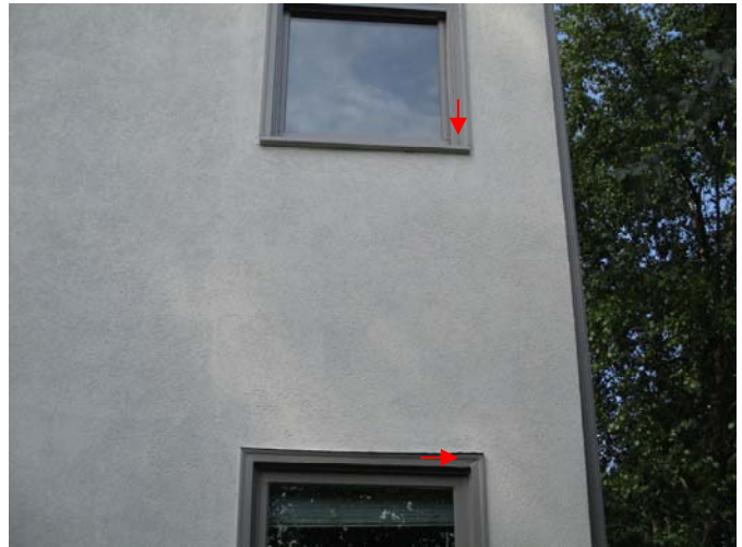
Moisture damage was present at the brick mould above the left side of the left window in the guest bedroom (main floor) and at the bottom of the brick mould on the left side of the left window in the back, left bedroom.
