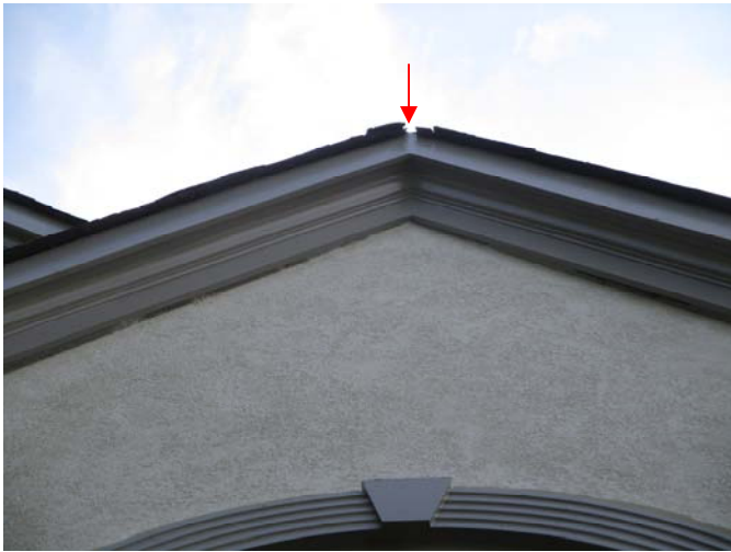
The shingle is cracked at the gable peak located above the window in the front wall of the foyer.
