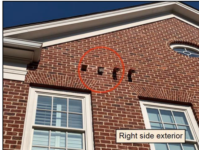
14. Screen on dryer vent
