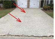
2. Walks: Concrete - Cracks present. A qualified contractor is recommended to evaluate and estimate repairs.
