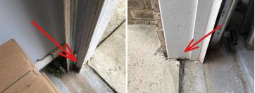
13. Front Garage Floor/Foundation: Poured slab - Items in garage covering floor and walls. Cracks present. A qualified contractor is recommended to evaluate and estimate repairs.
