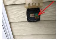
10. Vent: Plastic - Damaged vent. Recommend vent be repaired or replaced.
