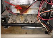
29. 3rd Floor Attic Heating System Blower Fan/Filter: Direct drive with disposable filter - Filter size 16 X 25 X 4. Filter is dirty. Recommend filter be replaced.
