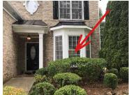
8. Exterior Lighting: Surface mount - Missing caulking around light fixtures. A qualified contractor is recommended to evaluate and estimate repairs.
