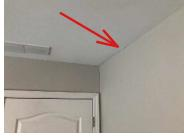
24. 3rd Floor Bedroom Ceiling: Paint - Cracks present. A qualified contractor is recommended to evaluate and estimate repairs.
