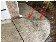
3. Patio: Concrete - Hairline crack present. A qualified contractor is recommended to evaluate and estimate repairs.
