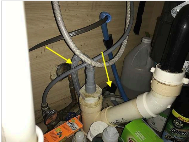
Dishwasher drain tube does not attach near countertop level
