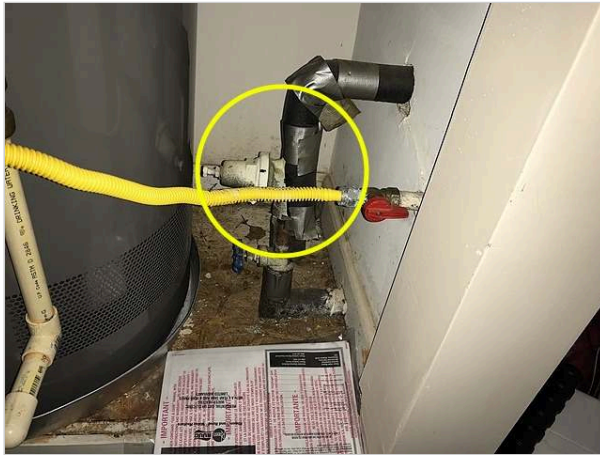
No bonding jumper
