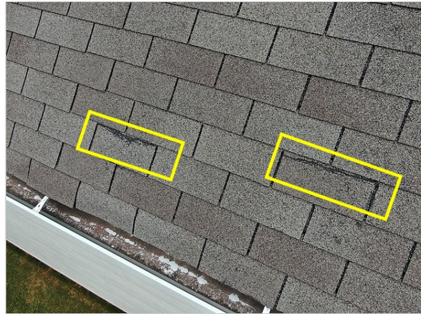
Possible wind damage
