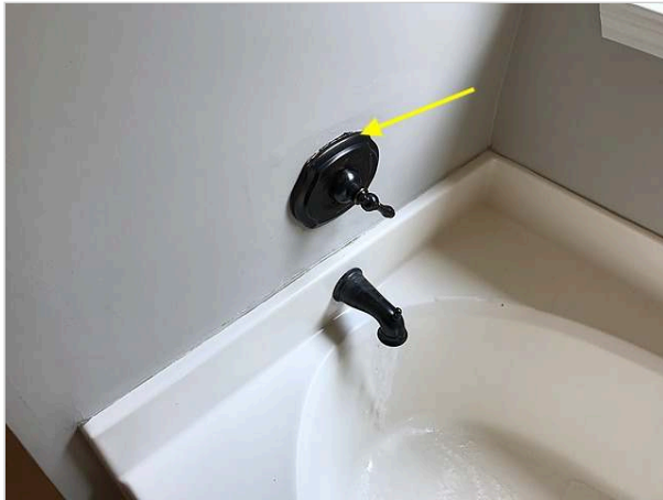
Fixture loose and not sealed to wall
