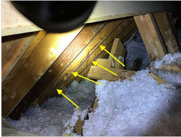
Moisture stains on attic framing
