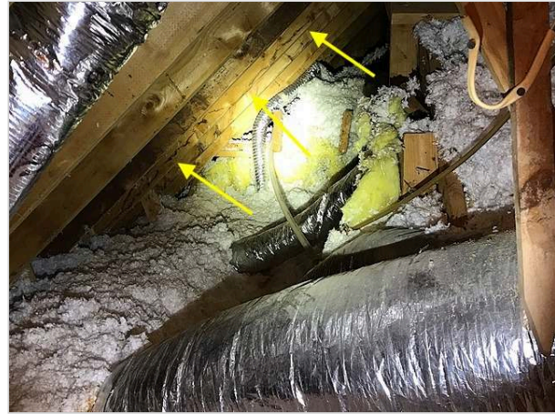
Moisture stains on attic framing
