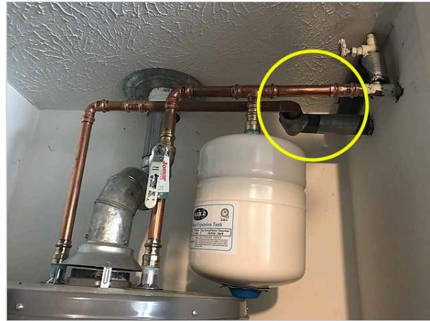
No bonding jumper
