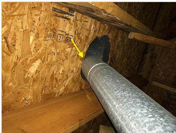
Furnace vent in contact with roofing material
