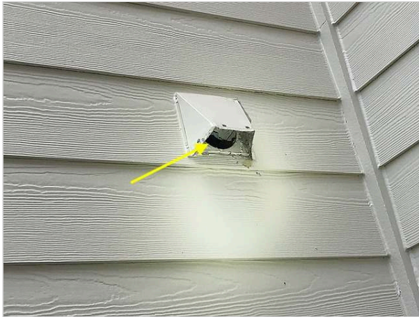
Missing rodent/insect flap at dryer vent
