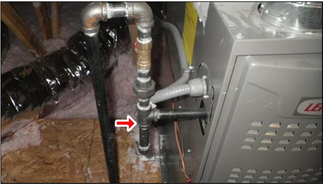
Proper sediment trap example
