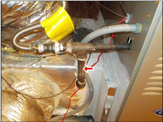
Existing, improper sediment trap
