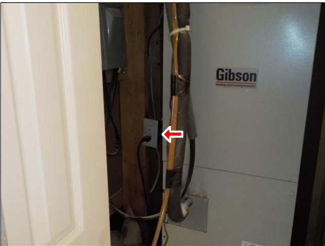
GFCI outlet next to air handler
