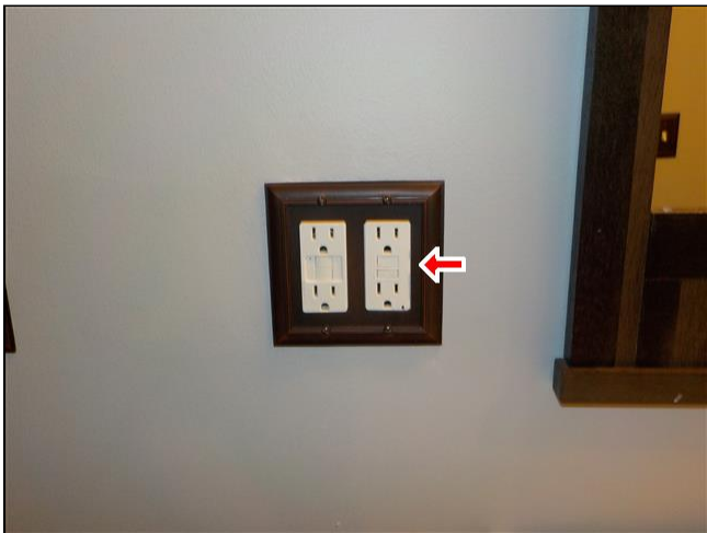
GFCI outlets in basement bath
