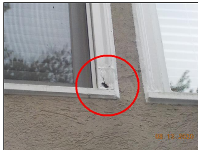
Wood rot and deterioration are present.
