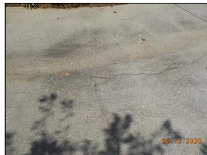
Recommended to seal all open cracks
