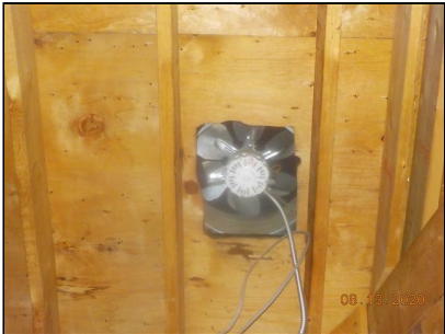
The attic roof power exhaust fan is not operating.
