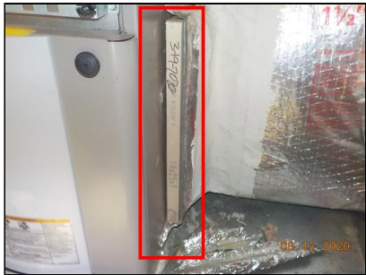
The filter access cover is missing.
