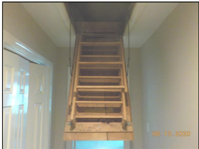
Attic pull down stair is not substantially weather tight when closed.
