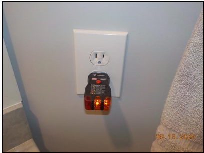
GFCI protection is missing.
