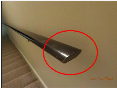
All hand rails should terminate back to a wall for safety
