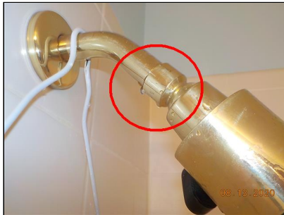
Leaking noted at the shower head connection
