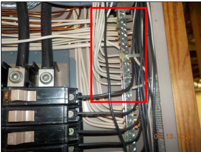
The neutral (white) wires are doubled under the same lugs
