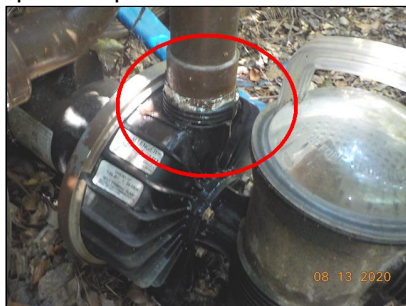
Leaking noted at the pool pump.
