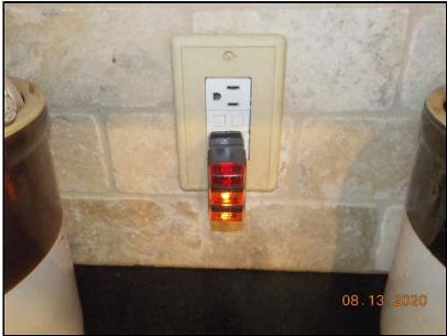
GFCI device failed to trip when tested
