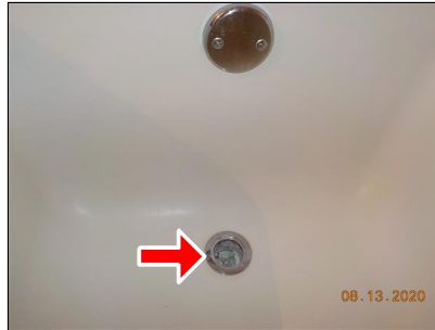
Tub stopper is missing
