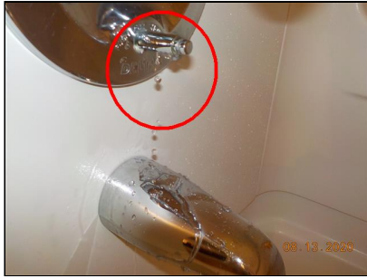
Shower diverter leaks when engaged.
