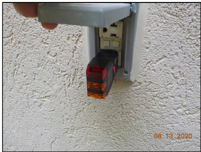
GFCI device failed to trip when tested
