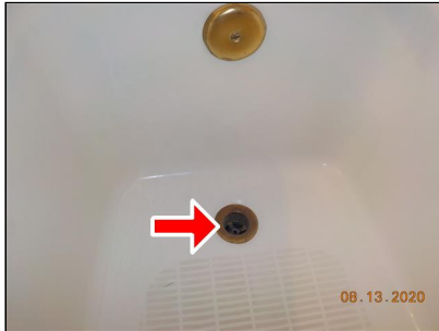
Tub stopper is missing
