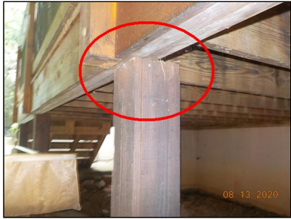
Support columns/posts are only toe nailed to the deck frame
