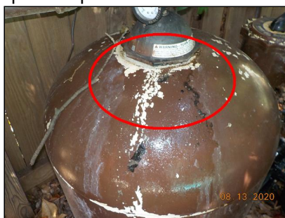
Leaking noted at the top of the filter.
