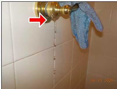
Faucet control valve stem leaks
