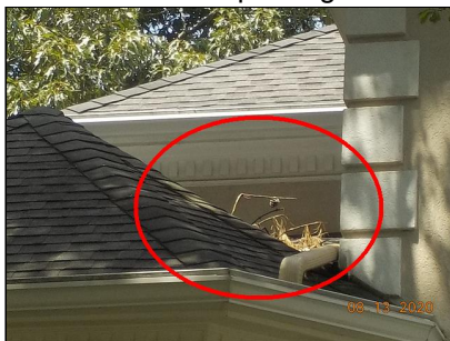
Organic debris (leaves, sticks, etc) is present on the roof covering.
