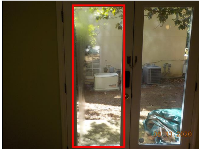
Condensation and / or hazing was noted between insulated window panes in glass door
