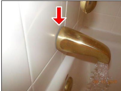
Fill spout is not tight to the tub wall.
