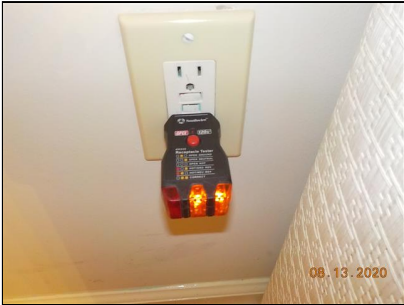
GFCI device failed to trip when tested
