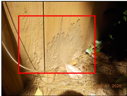
Termite damage noted.
