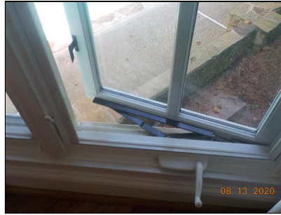
Windows crank out but do not crank back in
