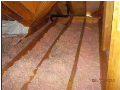
Visible ceiling joists means that thickness is less than 7 1/4 inches.
