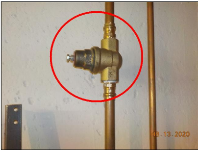
Adjustment/replacement of the pressure regulator valve (PRV) is necessary.
