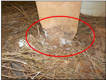
Wood rot noted at the base of the posts.
