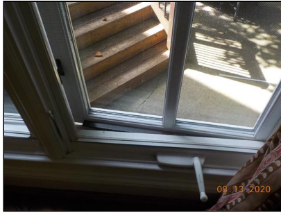
Windows crank out but do not crank back in
