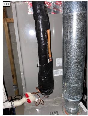
condensate line has a good slope Location Basement
