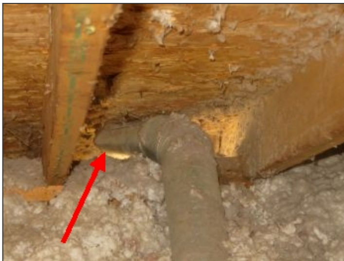
Dryer vent terminating in attic space
