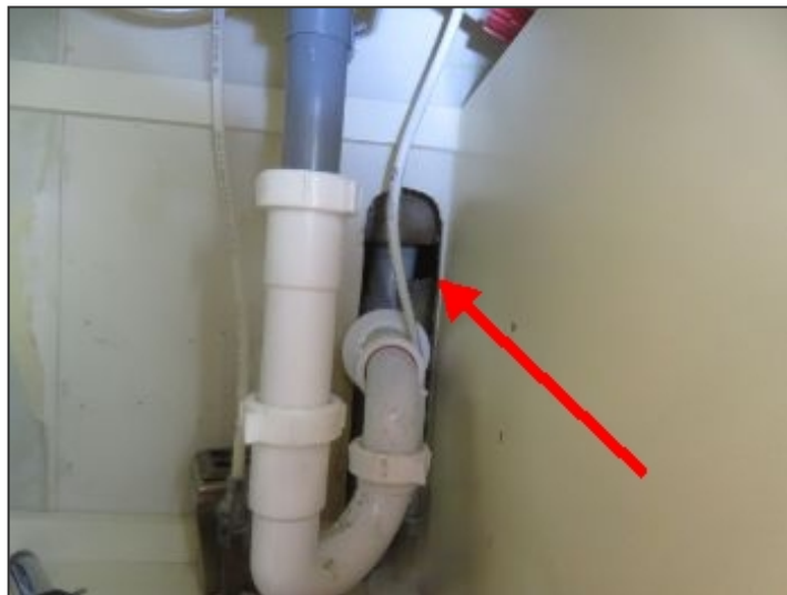
Opening into attic below second floor bathroom sink
