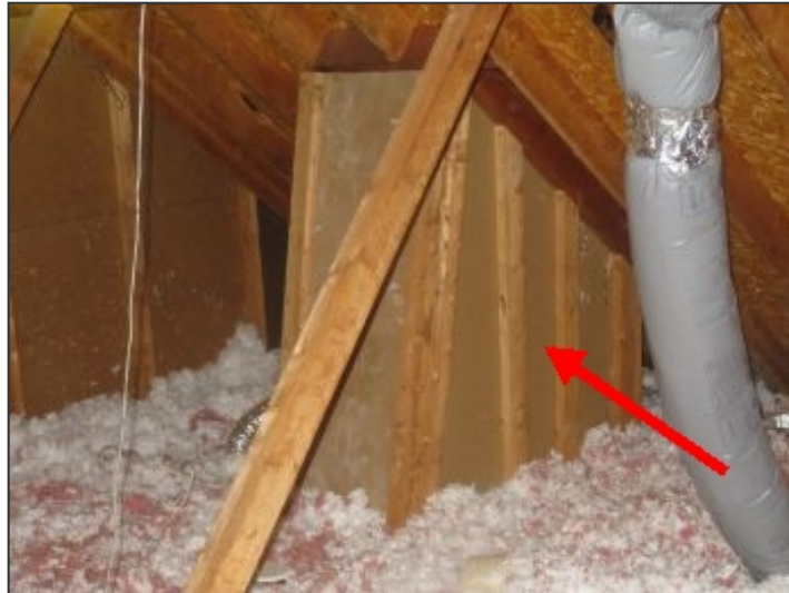
Missing insulation at vertical walls of skylight
