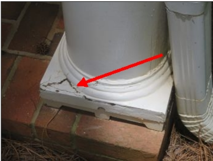
Damaged trim at front porch roof column
