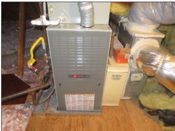
Gas furnace in attic
