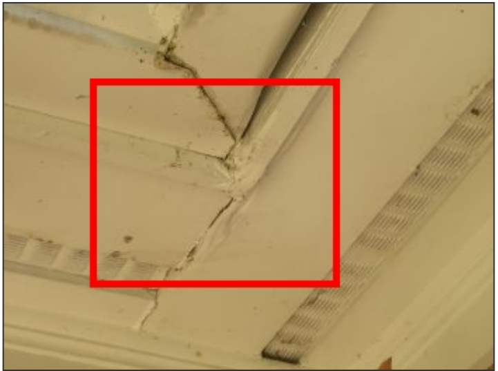
Damaged fascia and soffit at rear roof below chimney
