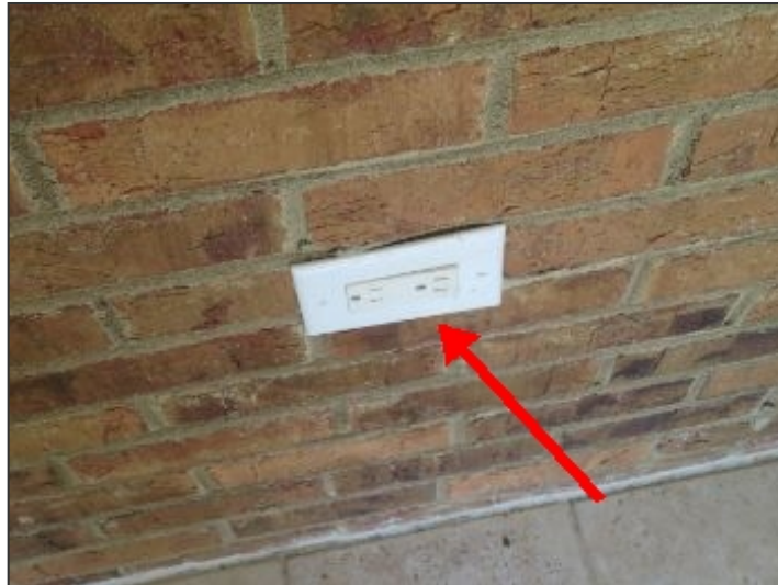
Screened patio outlet not weatherproof
