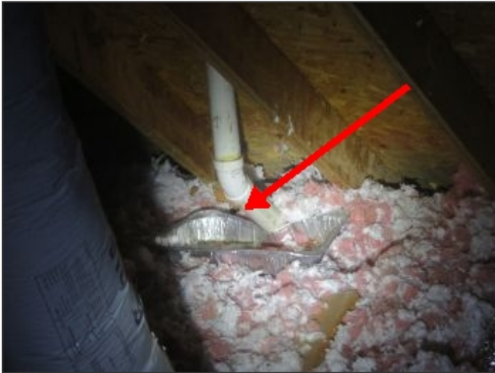
Container to catch leaks below master bathroom plumbing vent
