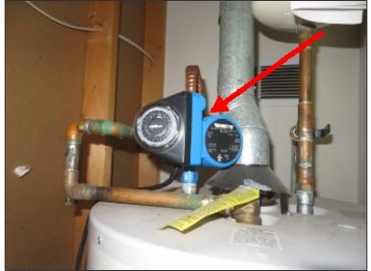
Recirculating pump at water heater
