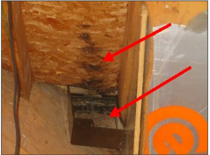
Water stains and container in attic at chimney
