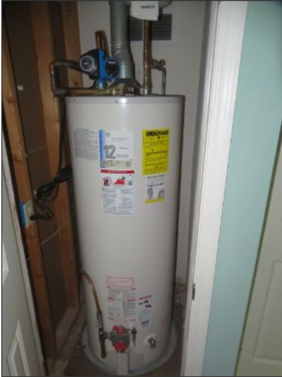
Gas water heater in bedroom closet
