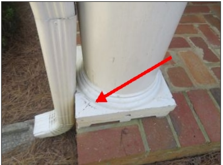
Damaged trim at front porch roof column
