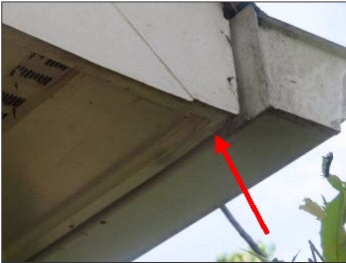
Damaged fascia at front left corner roof
