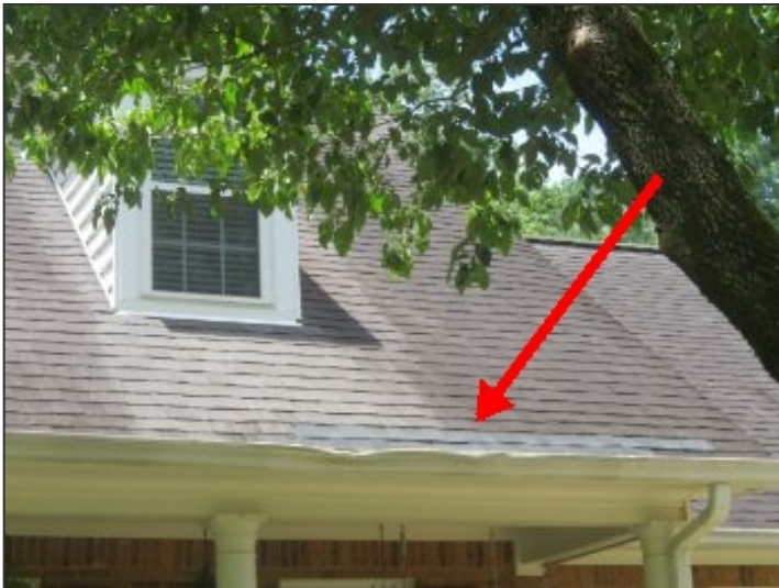
Shingle replacement at front roof
