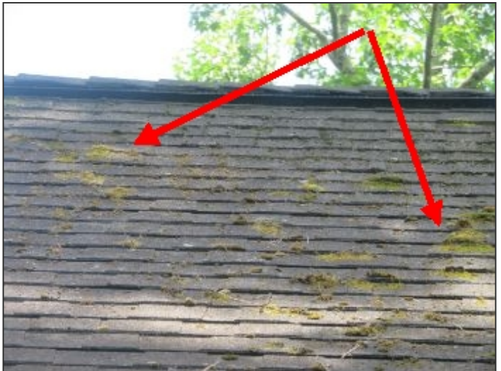
Excessive moss growth at front left roof
