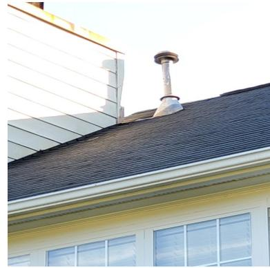
**5. REPAIR ROOF VENT IS NOT FLUSH WITH ROOFING. REPAIRED**
