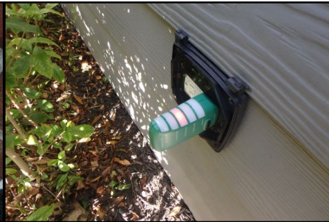
open ground on side exterior GFCI.*
