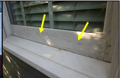
Peeling or missing paint, maintenance needed.*
