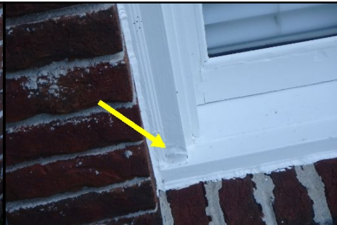
Decay or dry rot, repairs needed.*
