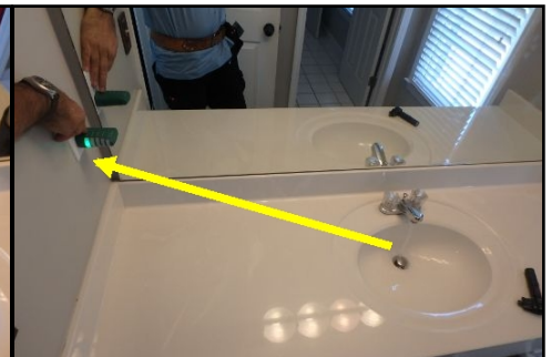
Recommend GFCI protection for bath outlets, missing in J&J bath.*
