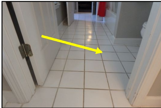
Floor is out of level in J&J bath.*
