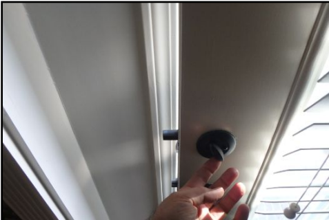
Dead bolt needs deeper hole to close properly at patio.*
