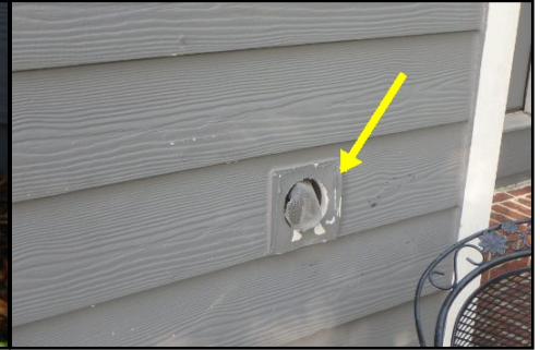
fireplace vent cover needs replacing.*
