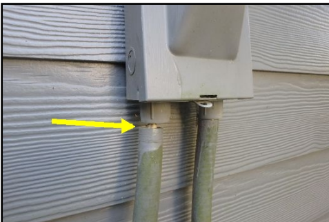
Loose conduit at AC unit needs securing.*
