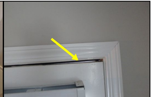
some exterior doors need weatherstrip, not lsealing.*
