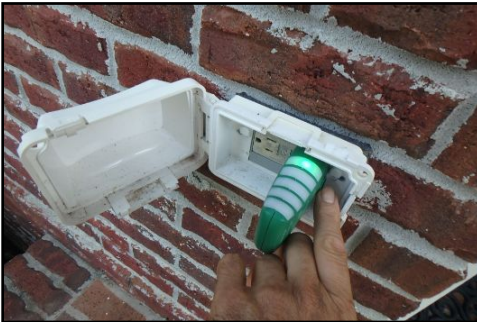
Most exterior GFCI outlets not tripping or not wired correctly.*
