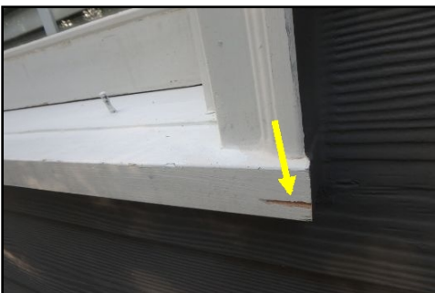
Peeling or missing paint, maintenance needed.*
