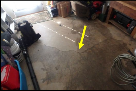
Common crack, not a concern
