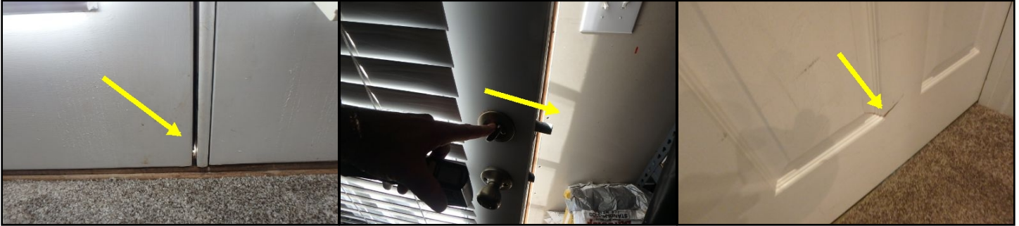
basement exterior doors not sealing well.*
