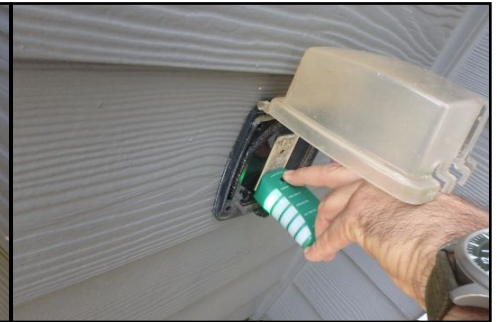
Most exterior GFCI outlets not tripping or not wired correctly.*
