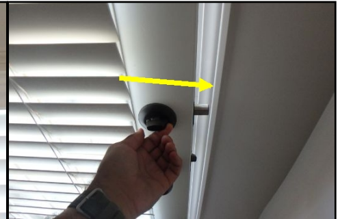
Dead bolt needs deeper hole to close properly at master.*
