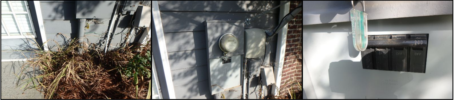
200 amp service, disconnect on right side
