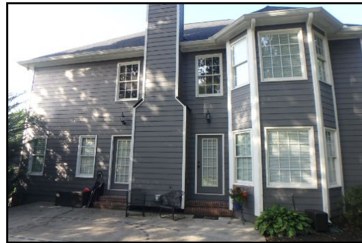
Grade is high at siding on right side.*
