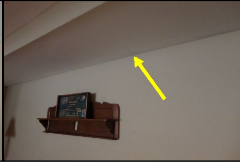
slight moisture present in basement ceiling under patio door.*
