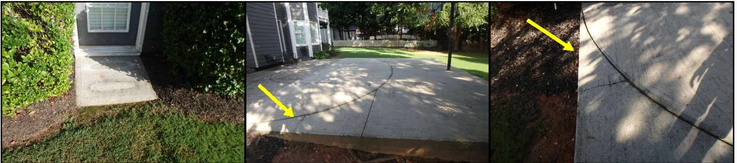
settling cracks at patio
