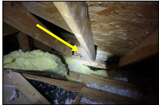
low insulation in master.*
