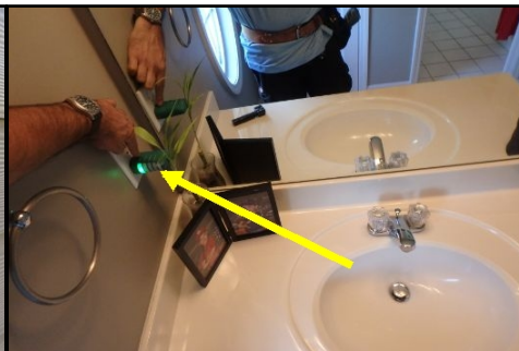
Recommend GFCI protection for bath outlets, missing in J&J bath.*
