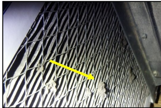
Filter needs to be replaced.*
