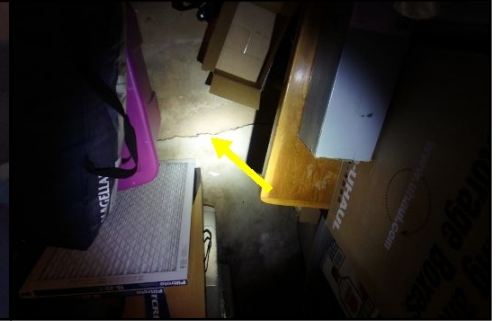
cracks in slab
