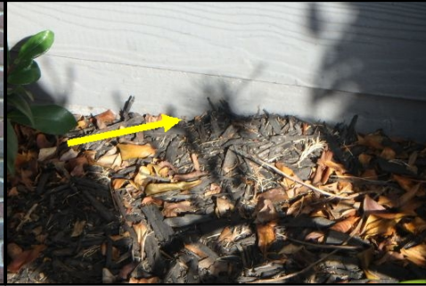
Grade is high at siding on right side.*
