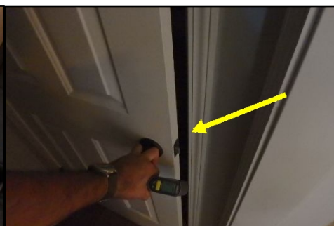
Door not latching, needs adjustment at coat closet .*
