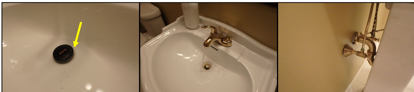
Slow drain in main floor bath sink.*
