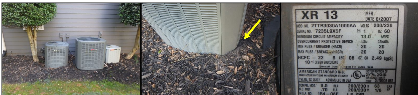
Recommend clearing debris at unit.*
