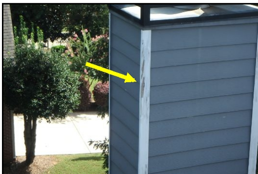
Peeling or missing paint, maintenance needed.*
