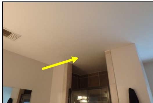
no light or exhaust fan in master shower.*
