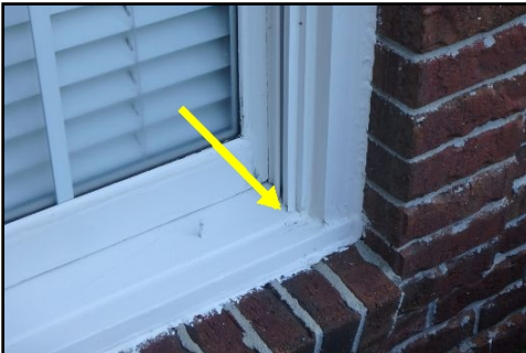
Decay or dry rot, repairs needed.*
