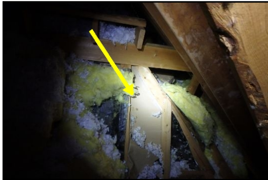
missing tray ceiling insulation.*
