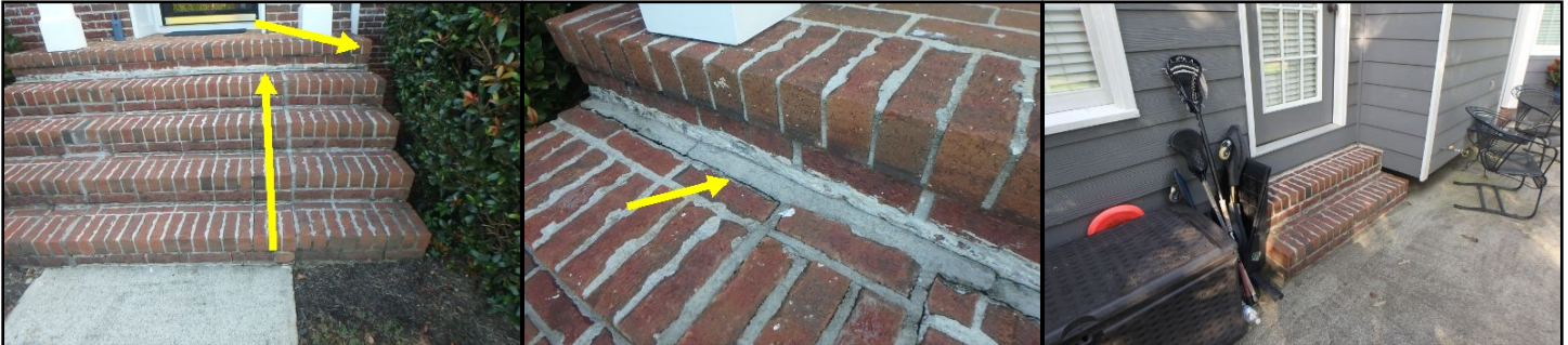
Settling and separation noted at entry steps, portion is out of level.*
