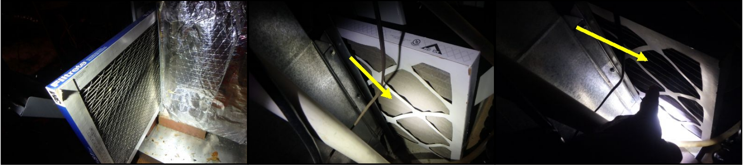
Filters need to be replaced in basement units.*
