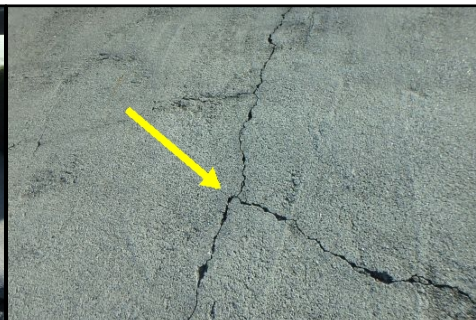
Common crack in driveway, not a concern.*
