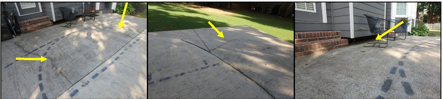
settling cracks at patio/court
