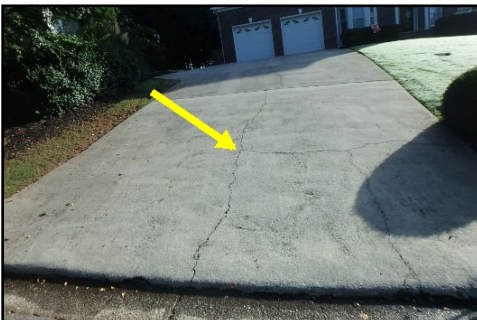
Common crack in driveway, not a concern.*
