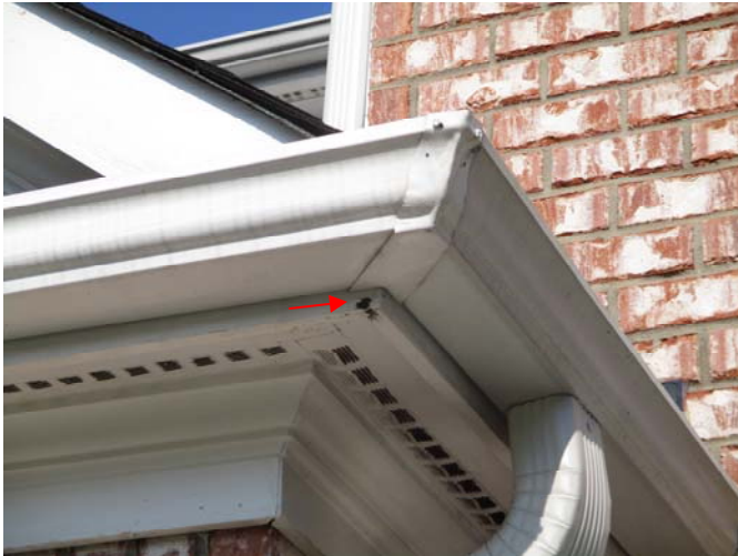
Moisture damage was present at the fascia boards below the corner joint in the gutter located above the right, front corner of the garage.
