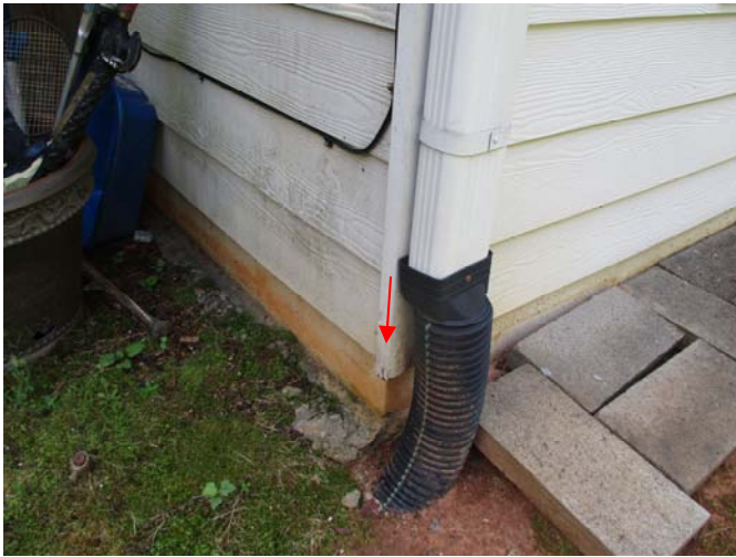
Moisture damage was present at the bottom of the corner trim at the back, right corner of the home.
