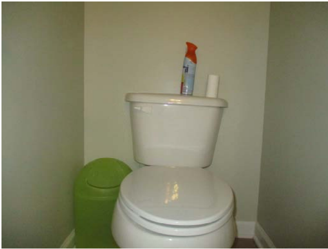
The tank on the commode in the master bathroom was installed at an angle, which is cosmetic in nature.
