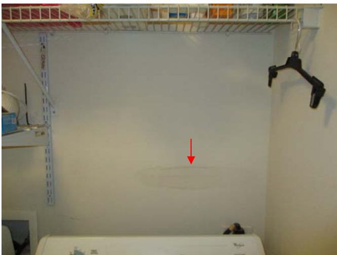
Inactive moisture stains were present on the wall above the backside of the dryer in the laundry room.
