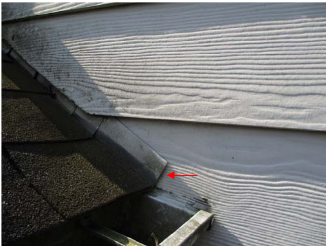
A licensed roofer or qualified contractor should install kick-out flashing under the last piece of roof flashing above the gutter on the left side of the chimney chase to prevent water from draining between the gutter and the siding during rains.
