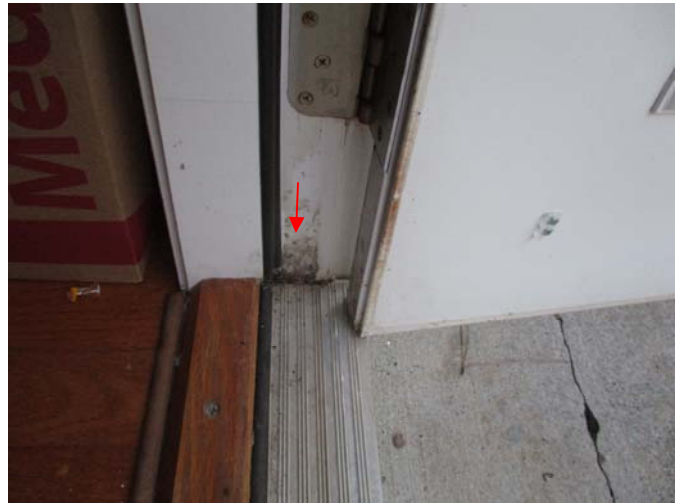
Moisture damage was present at the bottom of the frame on the left side of the left, exterior French door in the rear wall of the breakfast area.
