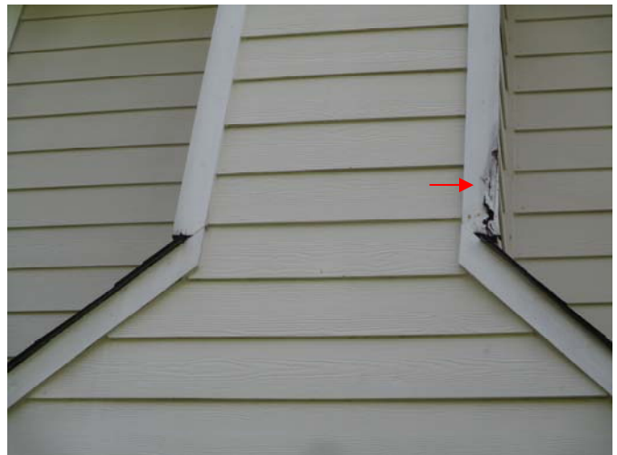
Moisture damage was present at the lower portion of the corner trim located above the small, shingled area on the right side of the chimney chase.
