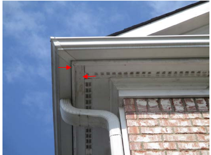
Moisture damage was present at the fascia and soffit boards located above the left, corner of the front, center bedroom.
