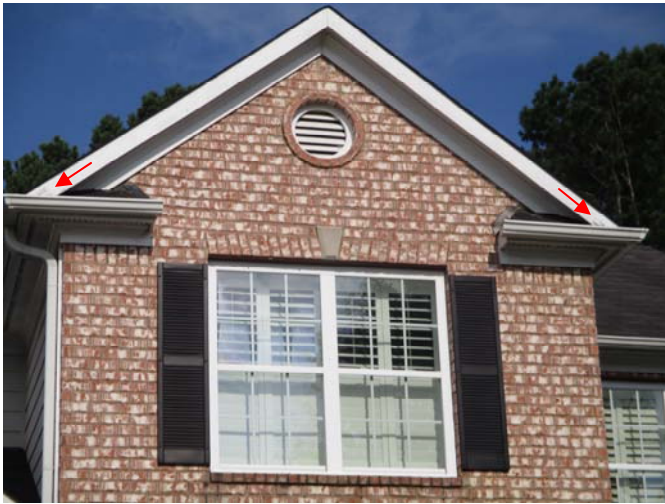
Moisture damage was present at the fascia board located below the right and left sides of the upper gable on the front of the home.
