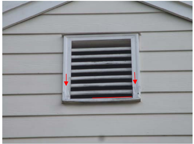
Moisture damage was present at the exterior trim located below the gable vent on the left side of the home.
