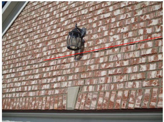
A qualified contractor should apply the missing mortar along the horizontal joint in the brick veneer cladding below the exterior light fixture located above the garage door.
