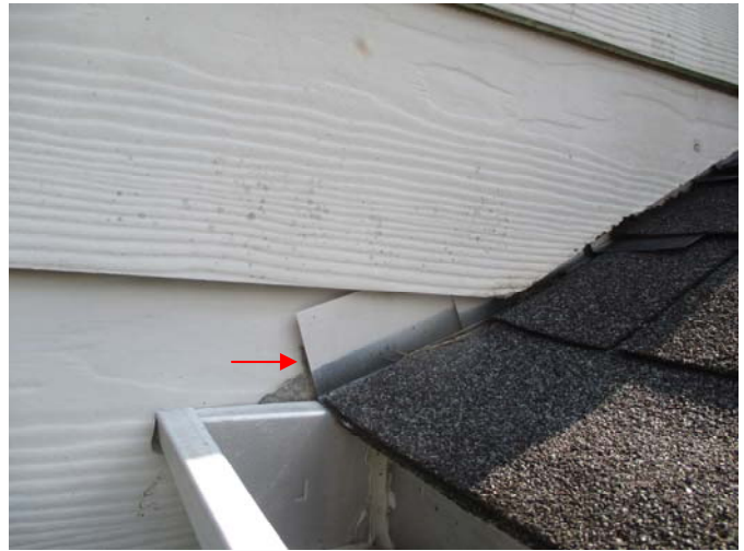
A licensed roofer or qualified contractor should install kick-out flashing under the last piece of roof flashing above the gutter on the right side of the chimney chase to prevent water from draining between the gutter and the siding during rains.
