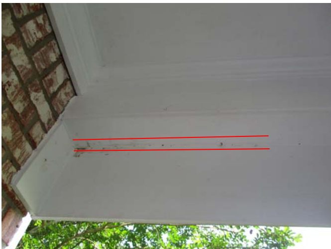
Moisture damage was present at the wood trim located under the right side of the front porch roof.
