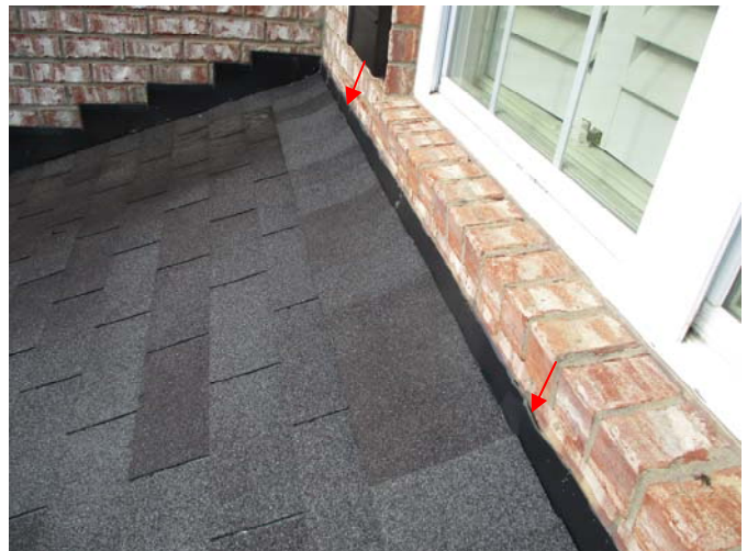
A qualified contractor should secure and re-apply the caulking along the top edge of the flashing located along the upper portion of the front porch roof to prevent future moisture entry.
