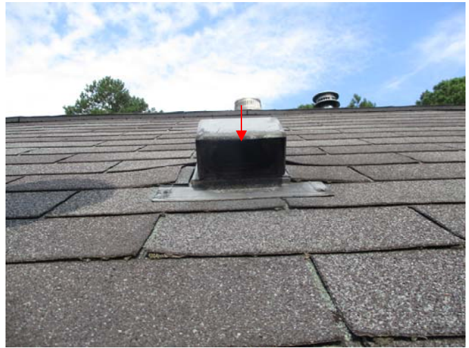
The dryer in the laundry room vents out through the shingles on the front of the home. The inside of the dryer vent and the venthood attached to the dryer vent located above the shingles should be cleaned by a qualified contractor.
