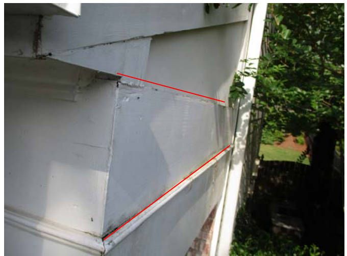
Moisture damage was present at the horizontal trim located above the right side of the front porch.
