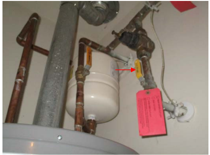
The shut-off valve on the main waterline is located above the right side of the water heater in the garage.
