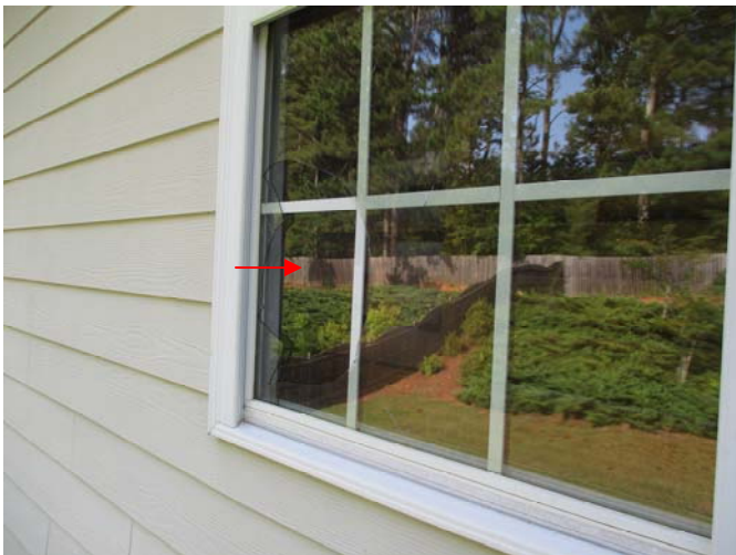
The lower piece of glass is cracked in the center window in the rear wall of the master bedroom.
