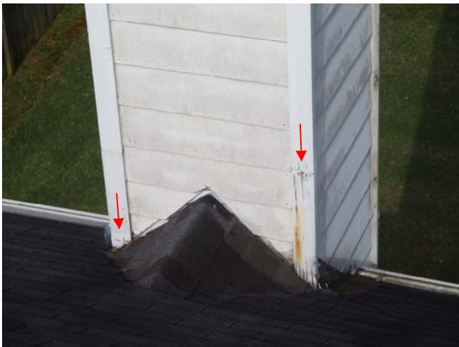
Moisture damage was present at the lower portion of the corner trim located at the back, right and left corners of the chimney chase.
