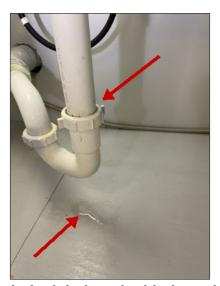
Drain leak below the kitchen sink
