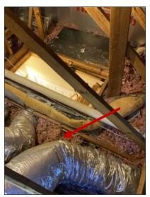
Missing walkway flooring to the furnace platform in the attic
