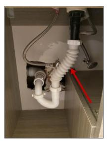
Improper flex drains below the master bathroom sinks
