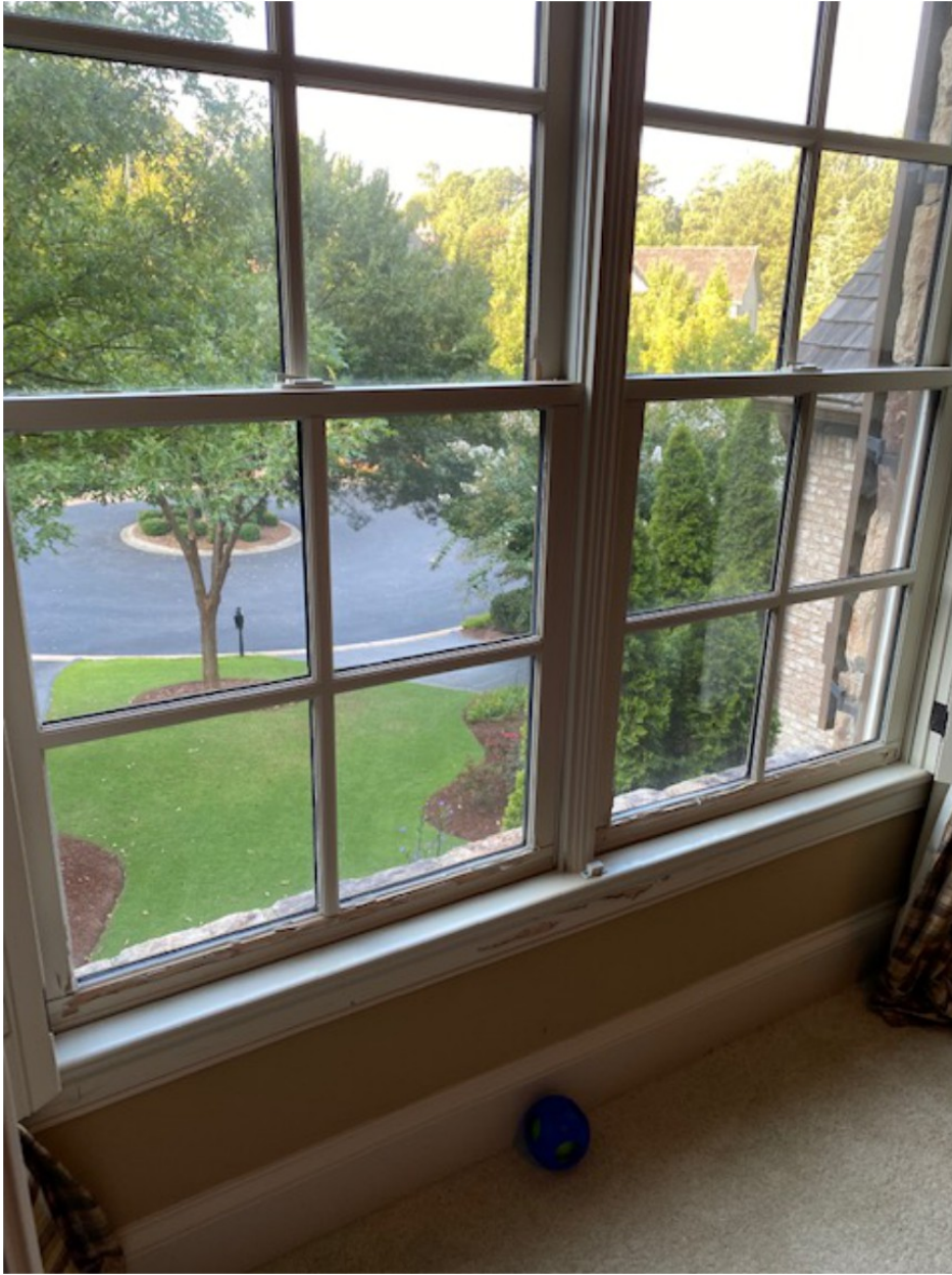
Seal, sand and paint
