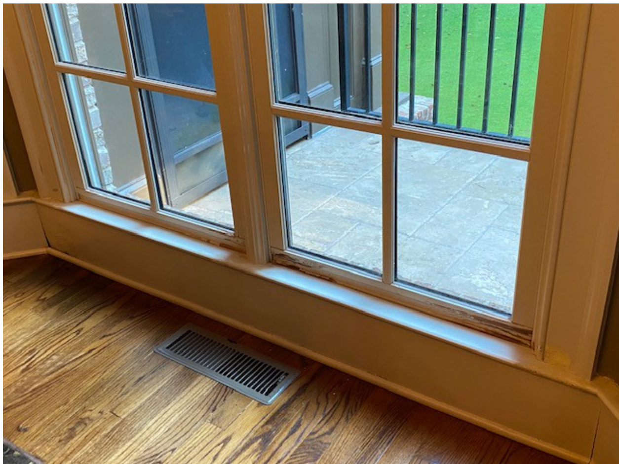
Seal, sand and paint
