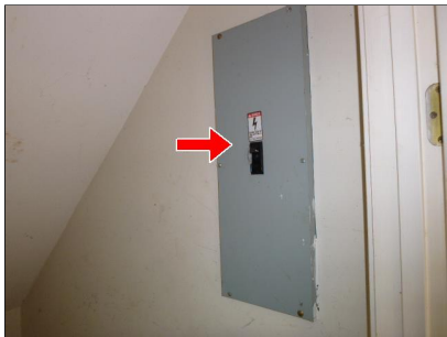
Main Breaker in Garage Closet
