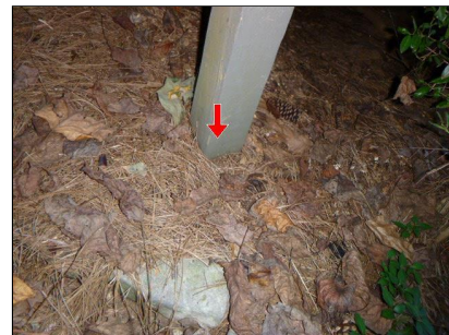
Posts in Contact with Soil
