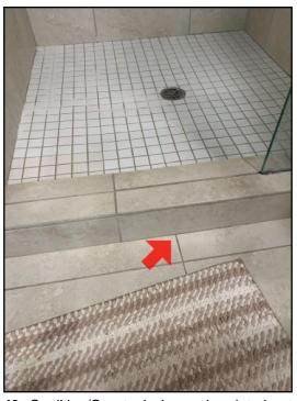
43. Caulking/Grout missing and or deteriorated
