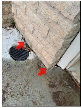
24. Drainage system for retaining wall is missing
