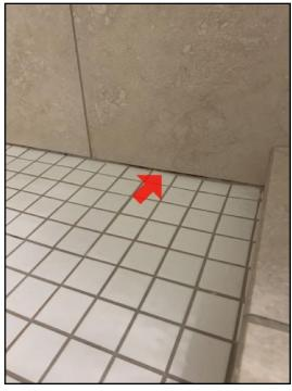
44. Caulking/Grout missing and or deteriorated
