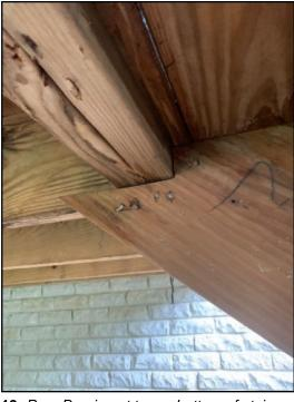
19. Poor Bearing at top or bottom of stair...
