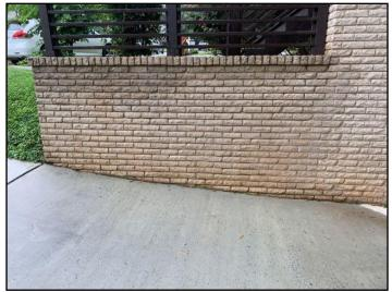
23. Drainage system for retaining wall is missing
