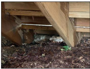
20. Poor Bearing at top or bottom of stair...
