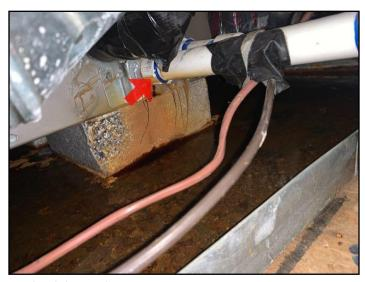
39. Leak in condensate system
