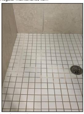
42. Caulking/Grout missing and or deteriorated
