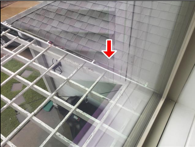
3.8 Gutter Holding Water
