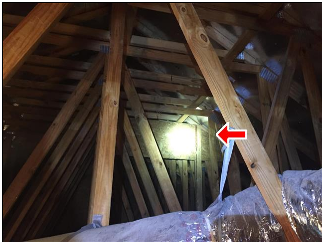
3.1 Damaged Truss
