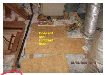
3.4 - The flooring from the access opening to the furnace should be continuous.
