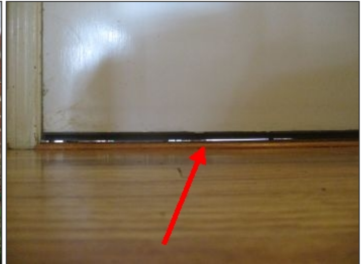
Threshold gap at garage entry door
