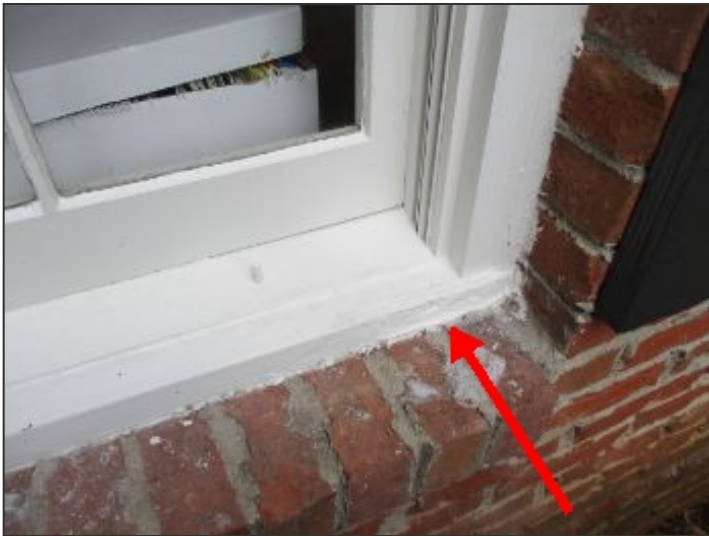
Damaged "nose" at office window sill
