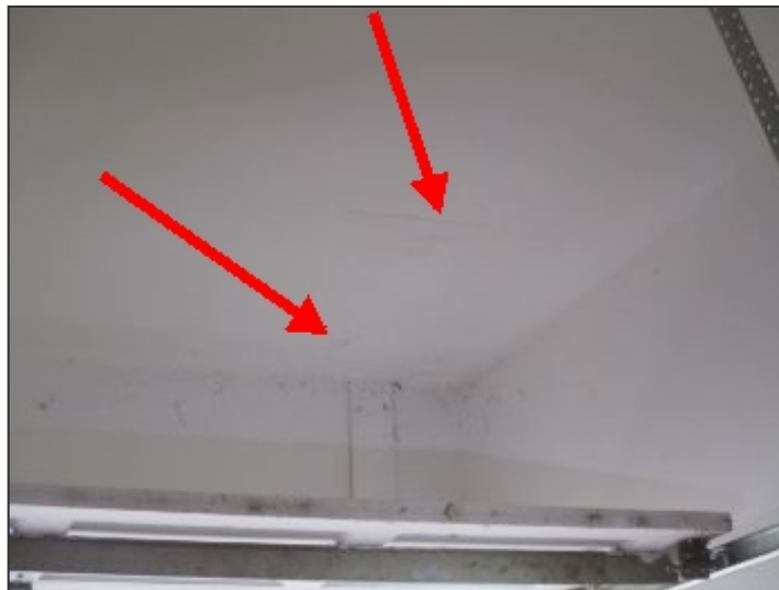
Water stain at garage ceiling
