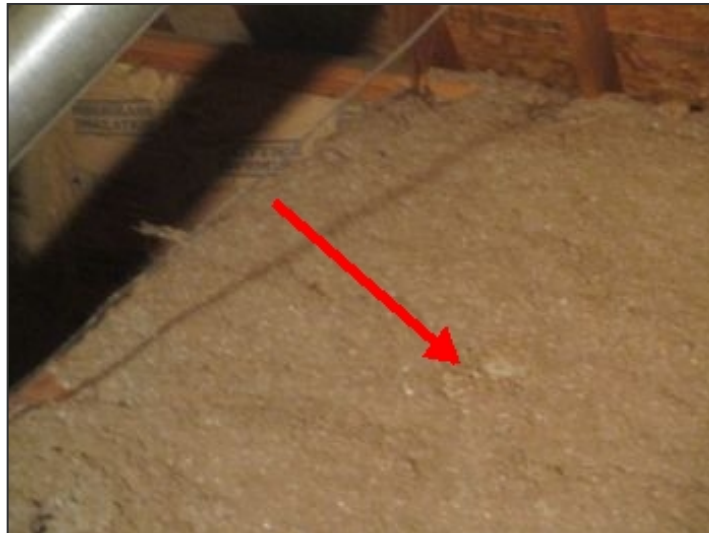
Water stain / divot in insulation below exhaust vent
