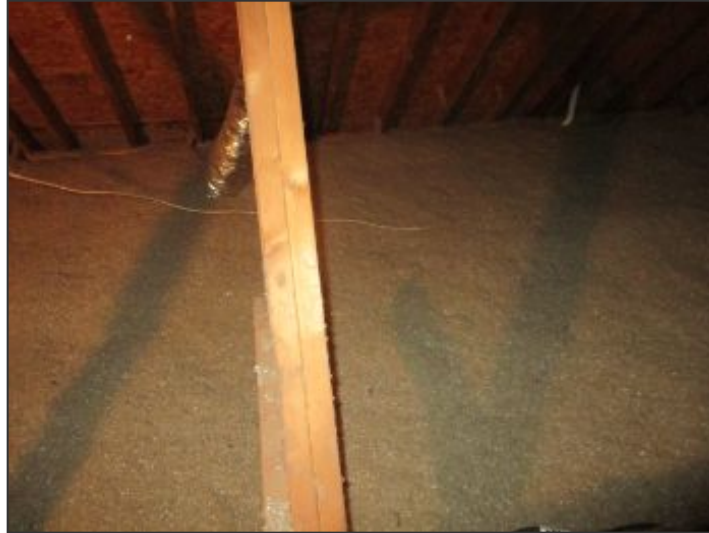
Insulation coverage in attic looks good
