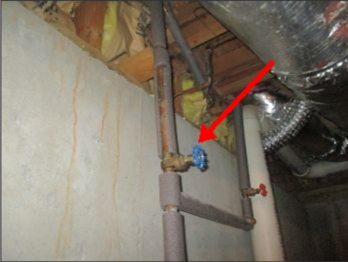
Main plumbing supply cut off valve
