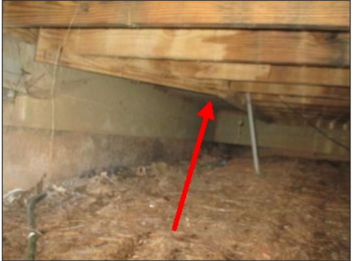
Deck attached to bay window / door
