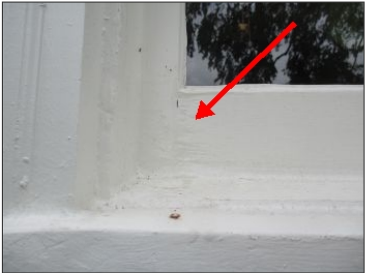
Damaged frame at living room window
