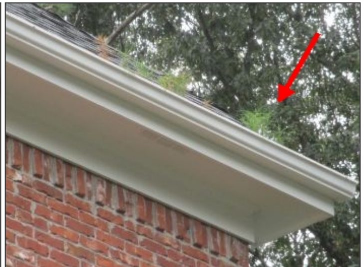
Debris in gutters at right side roof
