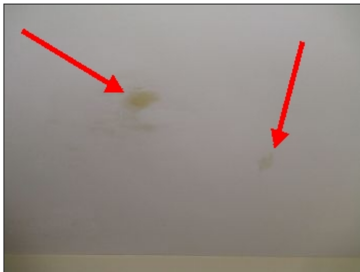
Suspected mold growth at basement ceiling below family room
