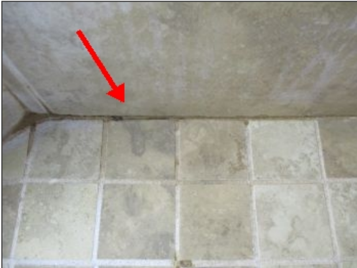
Openings in master bathroom shower grout
