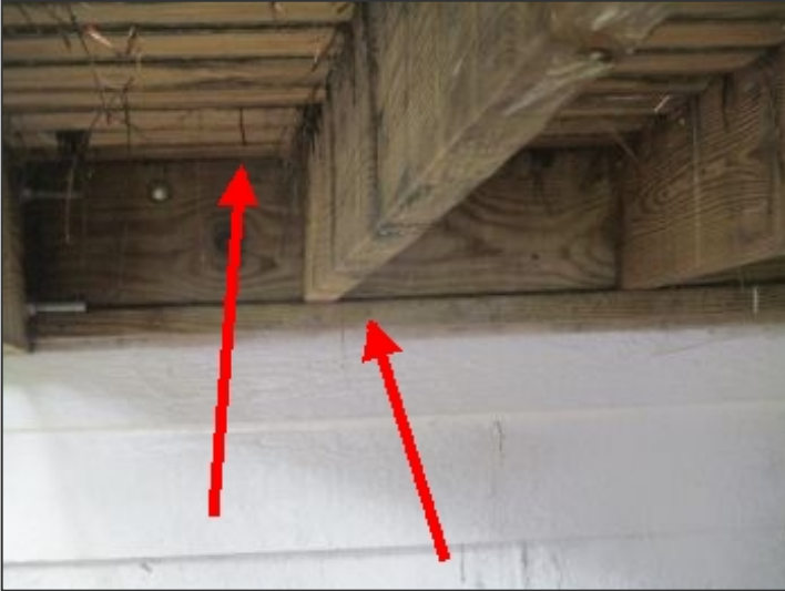
Missing flashing and joist hangers recommended at ledger board
