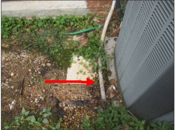
Good condensate drain extensions
