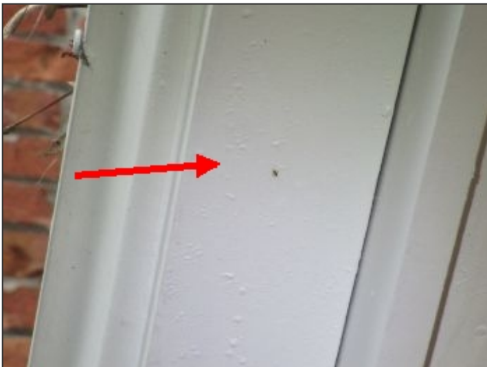
Corrosion staining at gutters
