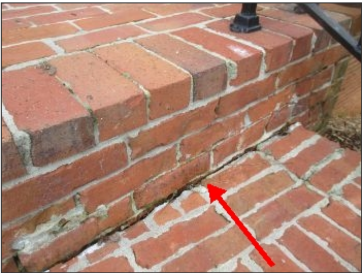
Settlement and separation at front porch stairway
