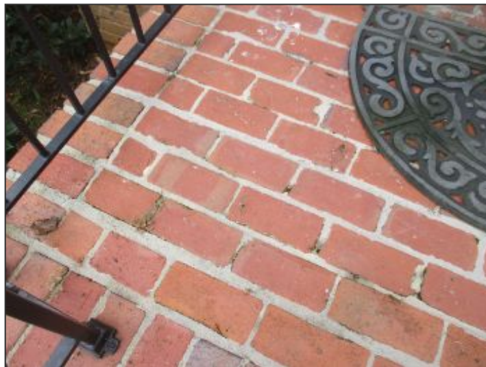
Deteriorating mortar at front porch
