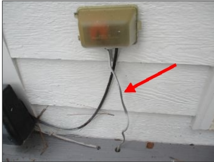
Missing conduit at rear deck extension cord
