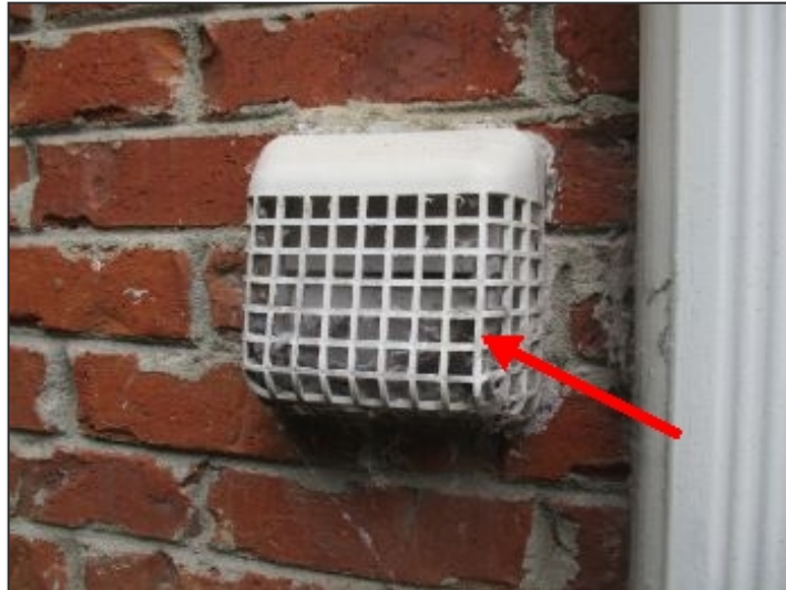
Screened dryer vent at exterior wall
