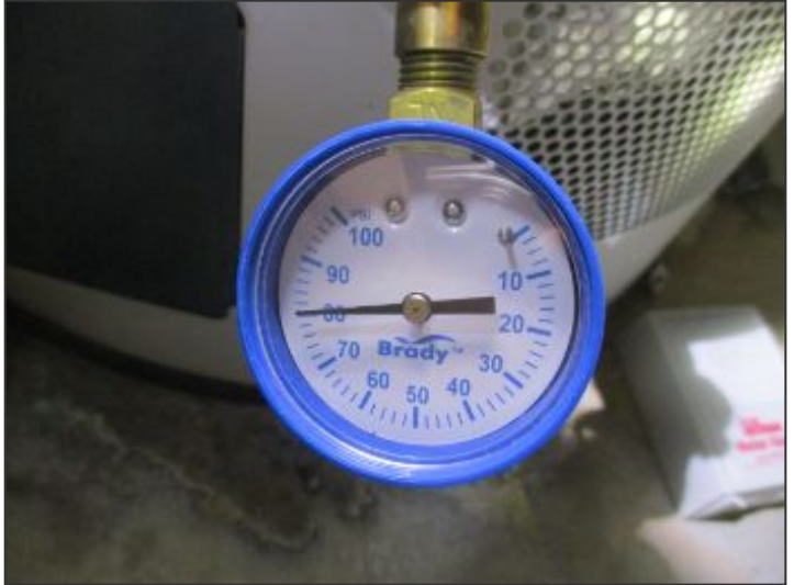
80 PSI normal at water heater
