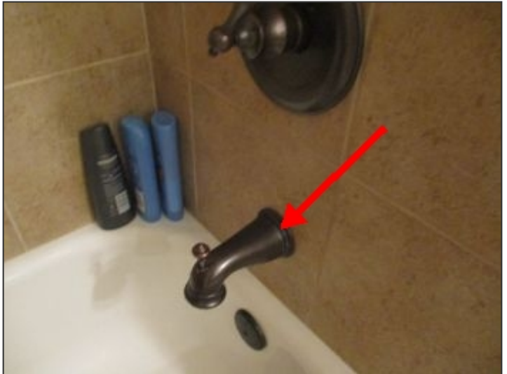
Unsecured faucet at basement tub
