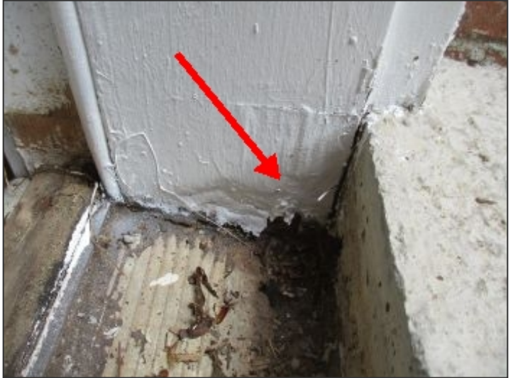
Damaged trim at basement side entry door
