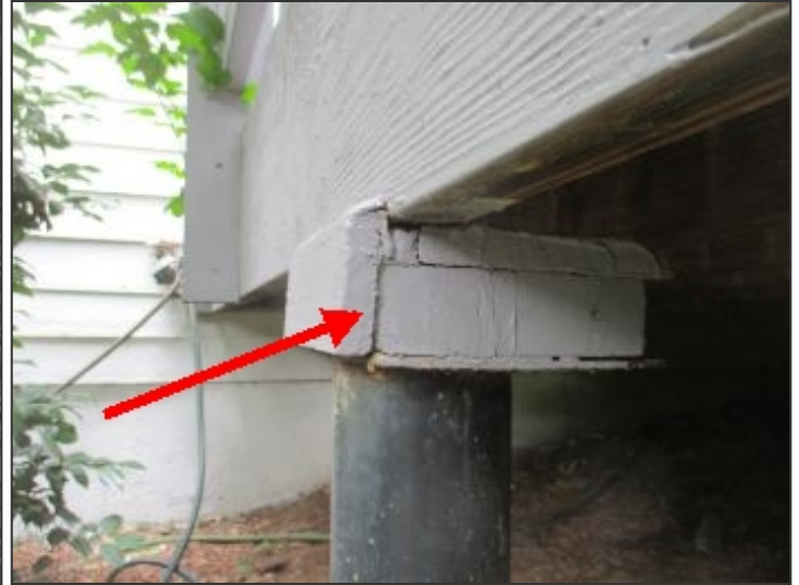
Wood shim at deck side rim joist
