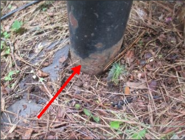
Deck support poles installed below grade
