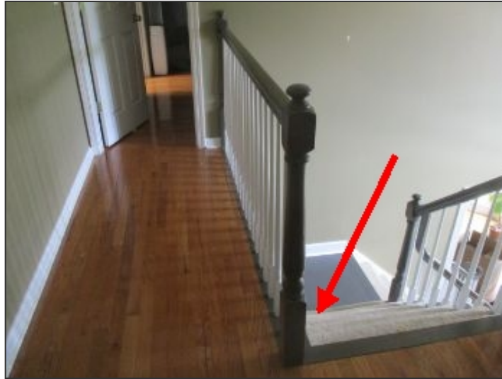
Loose guard rail at second floor hallway
