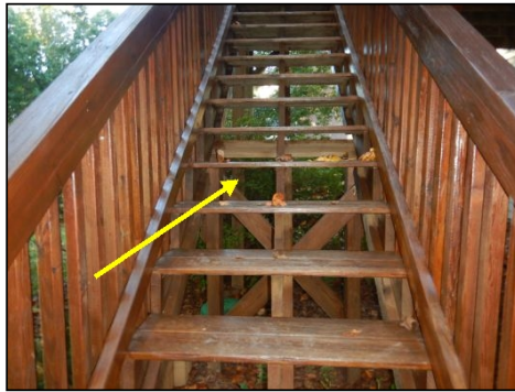
Open stair riser noted. No more than 4" between one tread to the next. This is a tripping hazard and child safety issue. This Does not apply to a total rise of 30" or less. Recommend review by qualified general contractor.
