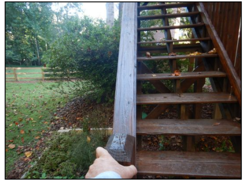
Noted the hand rails/stairs are loose. In the interest of safety, recommend repair by a qualified contractor.
