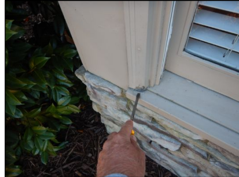
Moisture damage and wood rot noted. Recommend areas be addressed for repairs to include priming, painting and caulking by qualified contractor. front of home
