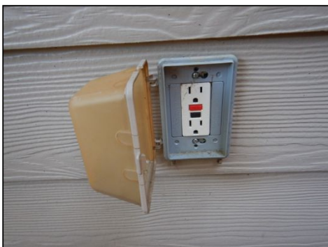
GFCI tripped when tested but would not reset. Recommend review or replacement by qualified electrical contractor. rear of home
