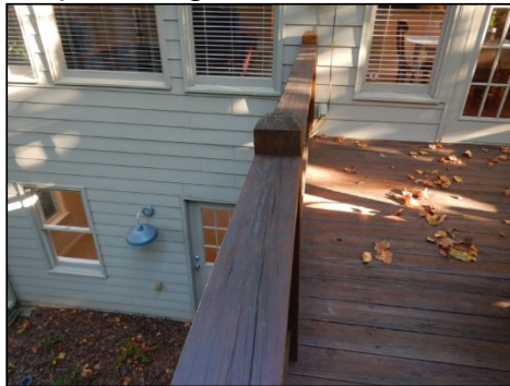
Noted the hand rails are loose. In the interest of safety, recommend repair by a qualified contractor.
