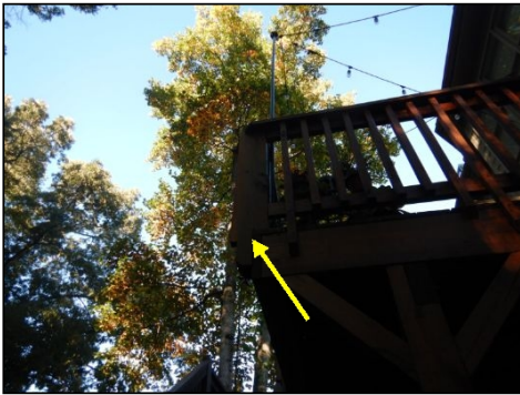
Improperly notched supports. Recommend review by qualified contractor.
