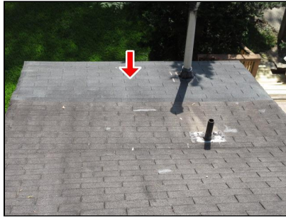
Rear Roof Above Laundry Room (Newer Shingles Noted)
