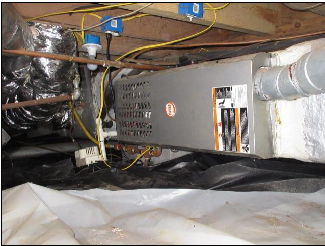
Gas Furnace (Located in Crawlspace)
