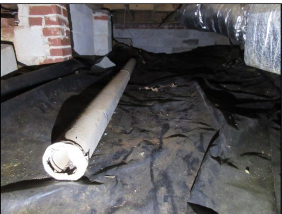
Vapor Barrier Noted in Crawlspace
