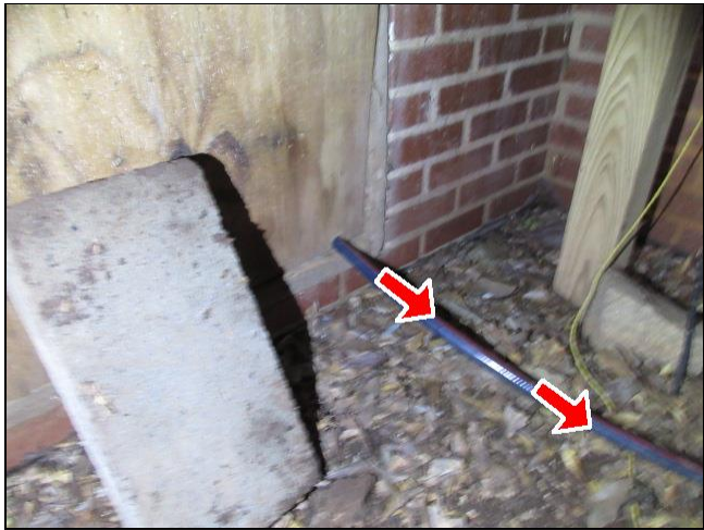
Hose Stretched Through the Crawlspace
