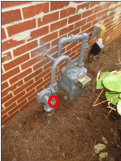
Gas Disconnect / Meter (Located at Left Yard)
