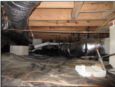
Floor Structure (Viewed from Crawlspace)
