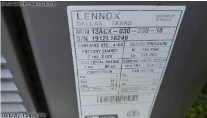
6.4 Air Temp Drop:     12 F Cooling not adequate. The temperature drop should fall between 14 and 21 degrees. The tested unit does not fall within this range. This could be the result of loss of refrigerant or poor operation on the equipment. Recommend repairs / replacement by a licensed HVAC technician.
