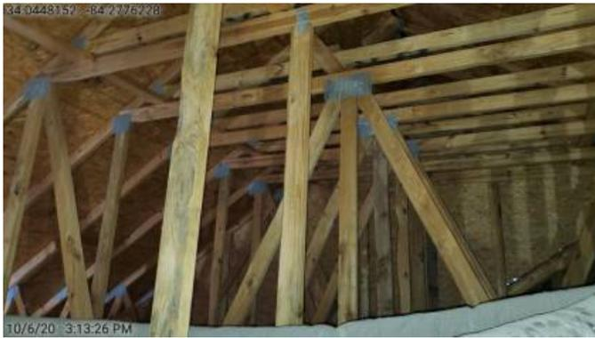
4.12 Structure Condition:     Repairs were noted to at least two trusses in the attic space around the first floor furnace. The repair on one section of the truss is loose and no longer effective. Recommend new Repairs by a licensed framing contractor.
