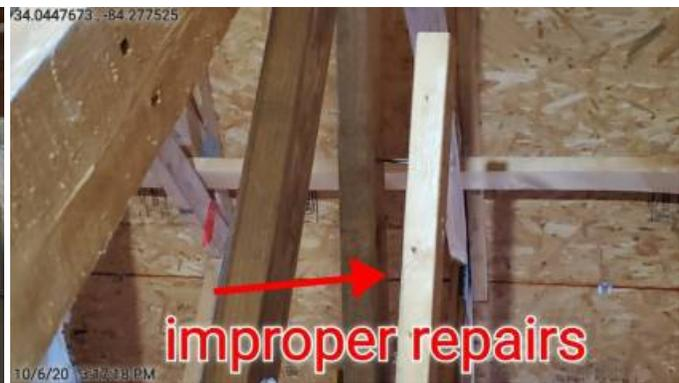
4.13 Moisture:     Dry water staining was noted on the framing. This appears to be from a previous leak on the roof.
