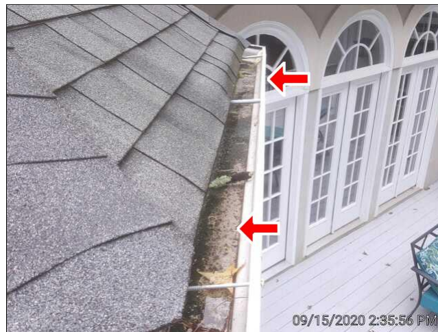
2.3 Item 1(Picture) water in gutters
