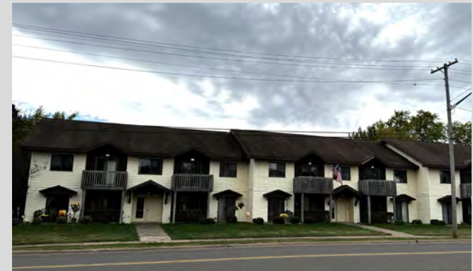
Multi-family housing across in Ironwood.
