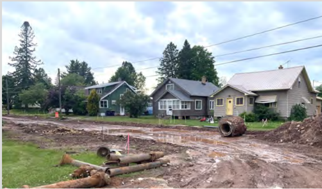
Ongoing improvements to replace aging pipes
