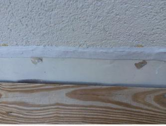
nail heads on the flashing are not sealed
