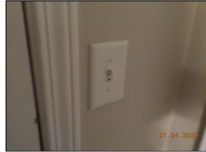
The second switch cannot turn the lights on from its position unless the dimmer is ON.
