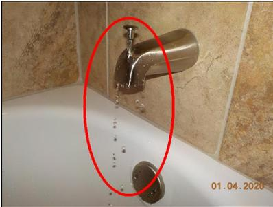
Shower diverter does not seal completely when engaged.
