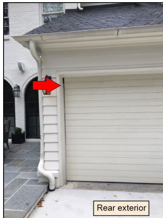
47. Weather Stripping Needed Task:...
