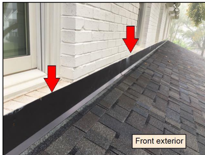
5. Caulking needed at seams Task:...
