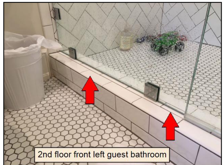
38. Caulking/Grout missing and or...
