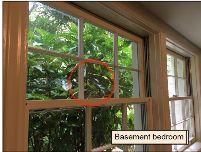
46. Cracked Glass Task: Repair Time: As Soon...
