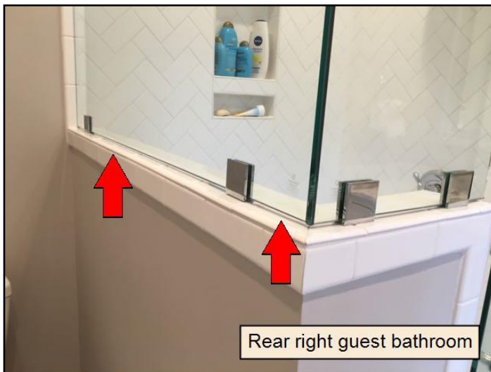
37. Caulking/Grout missing and or...
