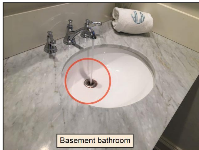
35. Drain stop missing
