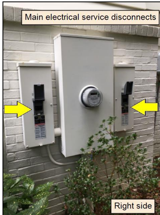
20. Breakers - exterior wall
