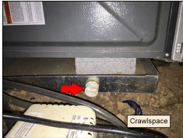
27. Missing cap / drain line
