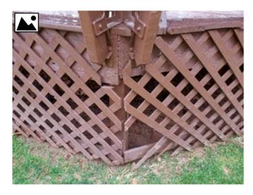
The beams are attached to the sides of the posts. This can effect the integrity of the structure. Issue Location Rear
