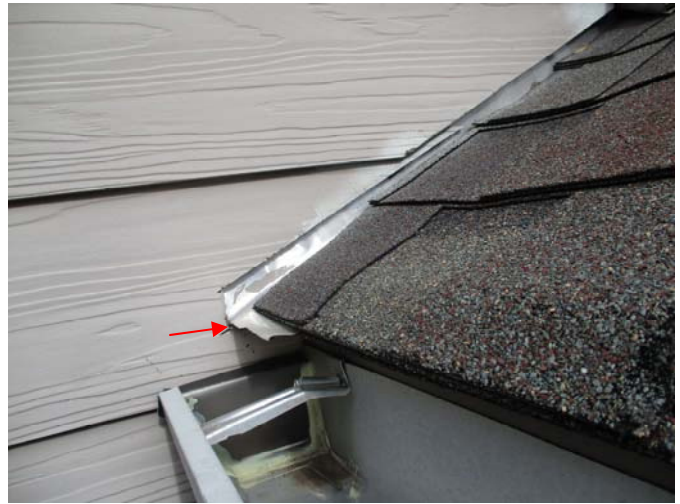
A licensed roofer should install kick-out flashing at the roof termination located above the gutter on the right and left sides of the chimney chase to prevent water from draining between the gutter and the siding during rains.
